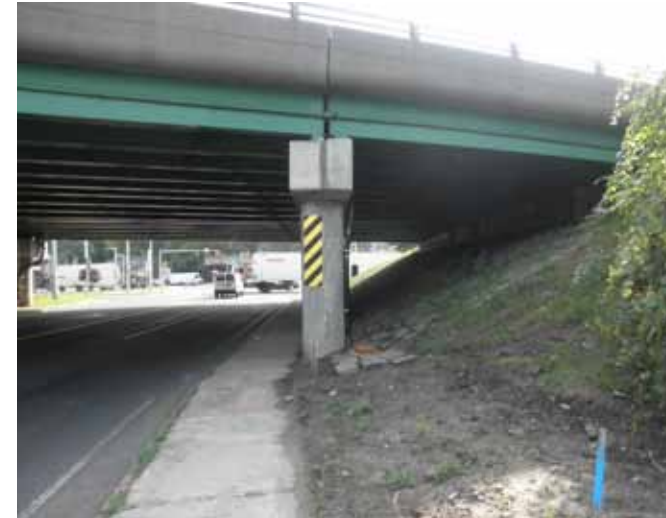
View Main Street underpass - existing conditions. The sidewalk is narrow.
