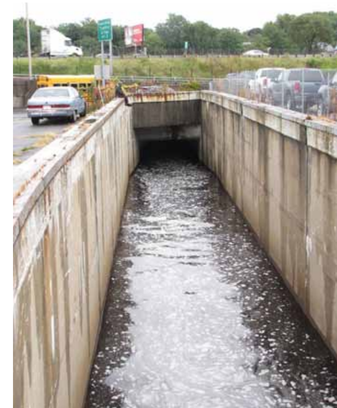
The culverted section of the Mill River is daylighted through the Balise property.
