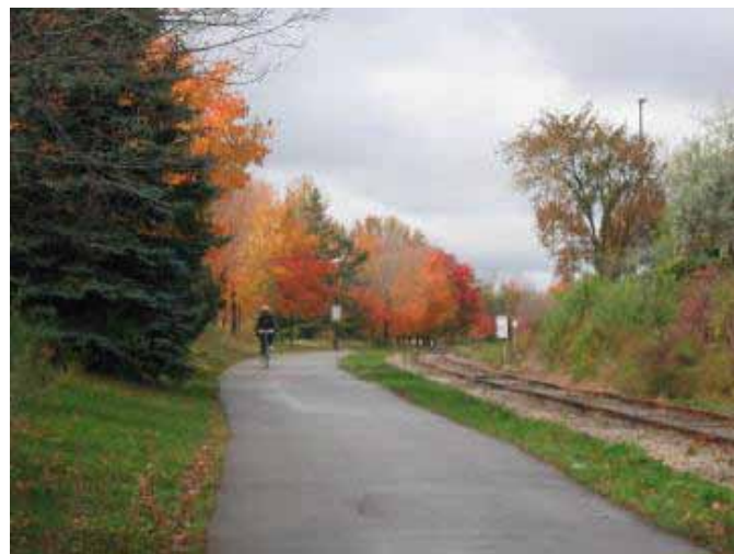
The need for fences is not necessary as pedestrians are kept a safe distance from passing trains.
