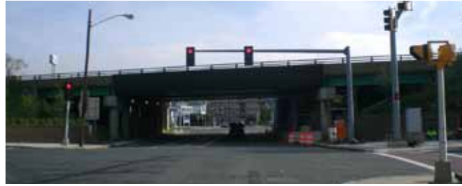
I-91 underpass at Broad Street facing Main Street
