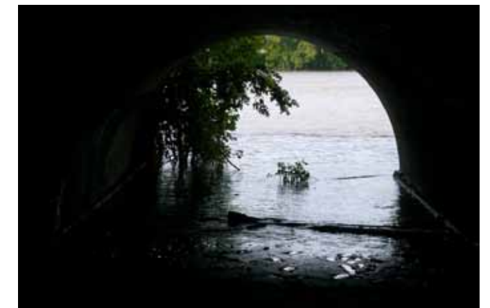
The Mill River joins the Connecticut River via a concrete culvert that runs underneath the city.
