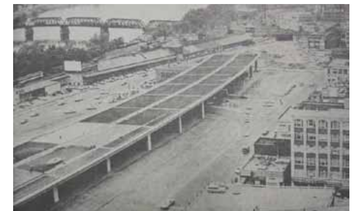
Construction of Highway I-91 in the early 1960's
