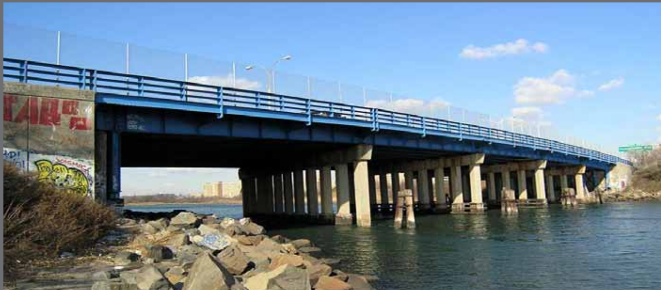
Existing Fresh Creek Basin Bridge
