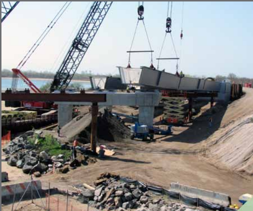
New Eastbound Paerdegat Basin Bridge under construction
