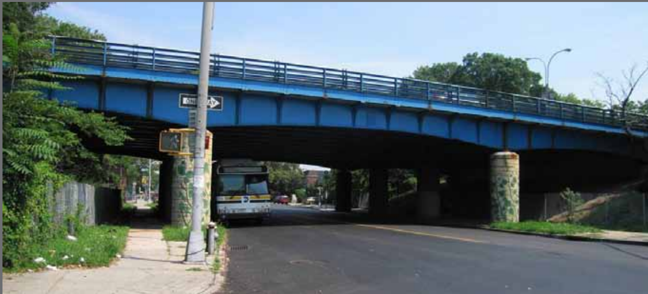
Existing Nostrand Avenue Bridge
