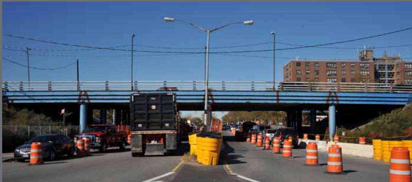
Existing Rockaway Parkway Bridge under construction
