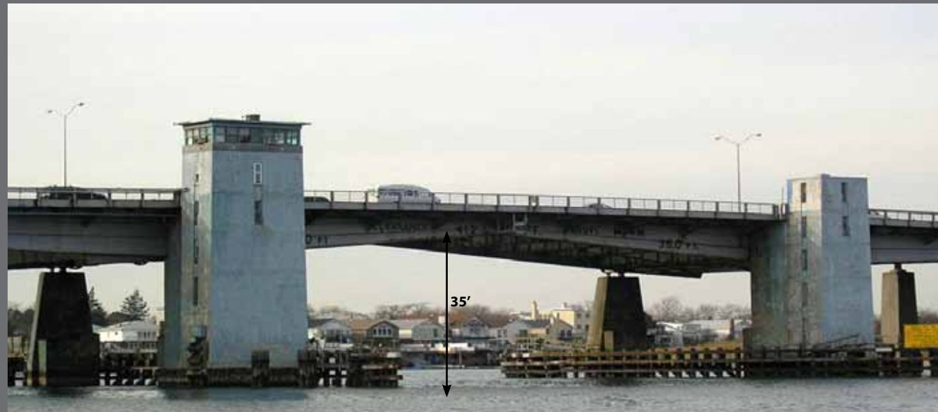
Existing Mill Basin Bridge
