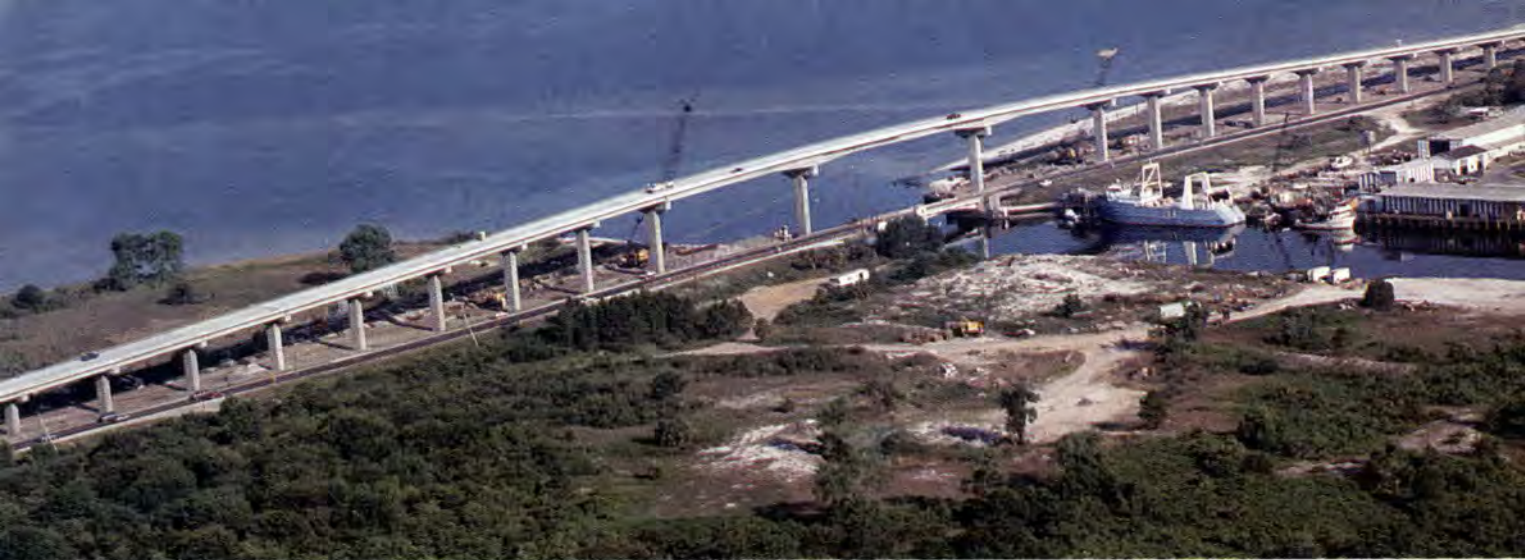
Fig. 13. Aerial view of completed Highland View Bridge.
