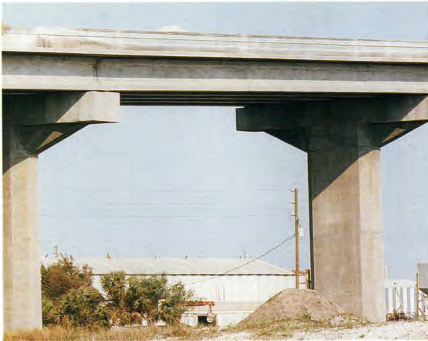
Fig. 6. Closeup view of octagonal columns showing tapering pier cap.
