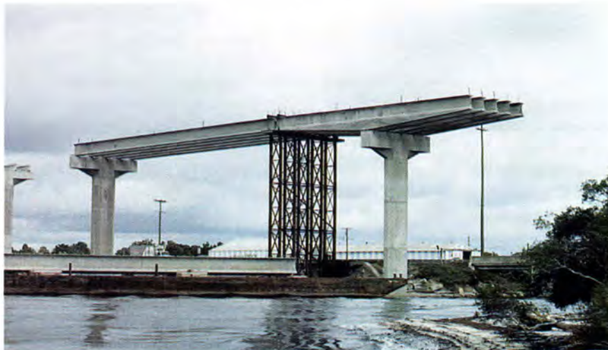
Fig. 12. Completion of span adjacent to main span.
