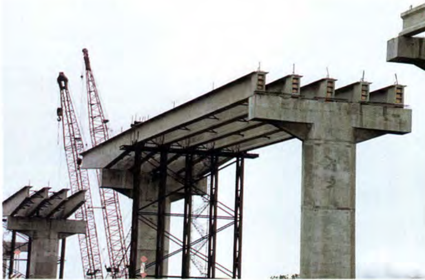
Fig. 11. Erection of end spans over piers.
