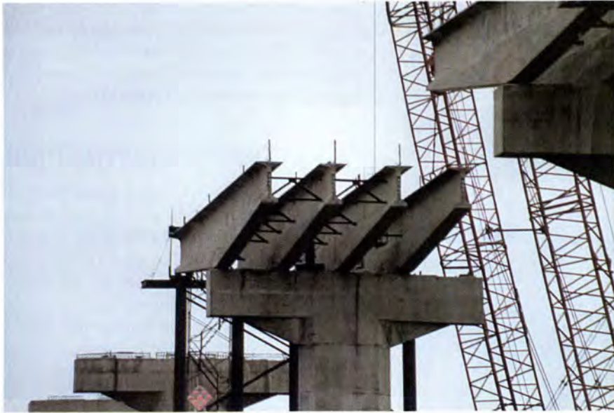
Fig. 10. Installation of haunched girder sections over piers.
