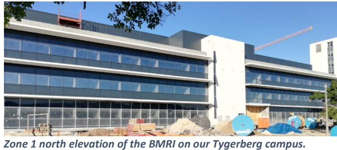
Zone 1 north elevation of the BMRI on our Tygerberg campus.
