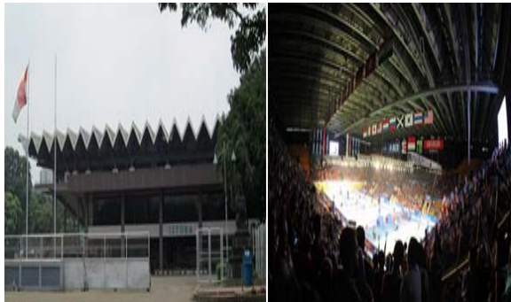
Figure-15. The exterior and the interior of Istora Senayan showing the folded roof [21] and its steel frame structure [22].
