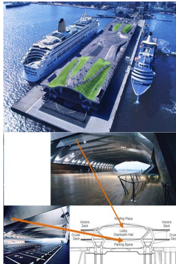
Figure-13. (top): Yokohama Port Terminal [18]; (centre): Lobby/Osanbashi Hall; (bottom left): Parking Space; (bottom right): A Cross Section of the Port Terminal showing the location of the origami ceilings.
