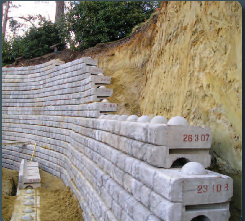
Redi-Rock dome and groove joint
