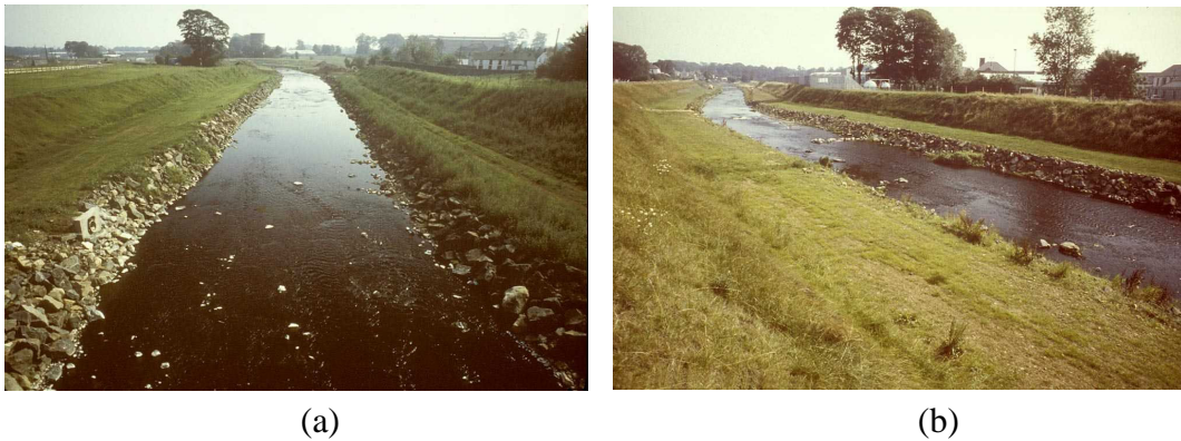
Figure 6.4 River Main in County Antrim, Northern Ireland (a) the cobbled side-banks and (b) a gentle meander
