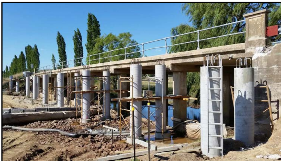
Bergen Bridge Widening Project in progress – Project completed June 2017
