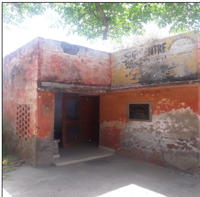
Figure 5: Two room Primary Health Centre of Village Suchetgarh (© Author)
