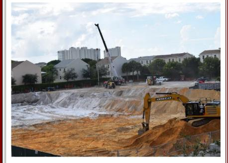
Steel sheet piles, a vertical interlocking system that creates a continuous wall, are in place and more than a quarter of excavating is finished
