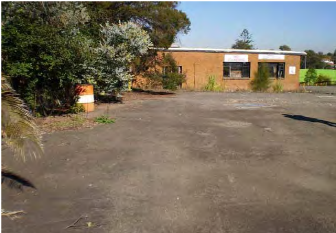
Photo 36 - Former Global TV garage building at south-eastern boundary of site facing east
