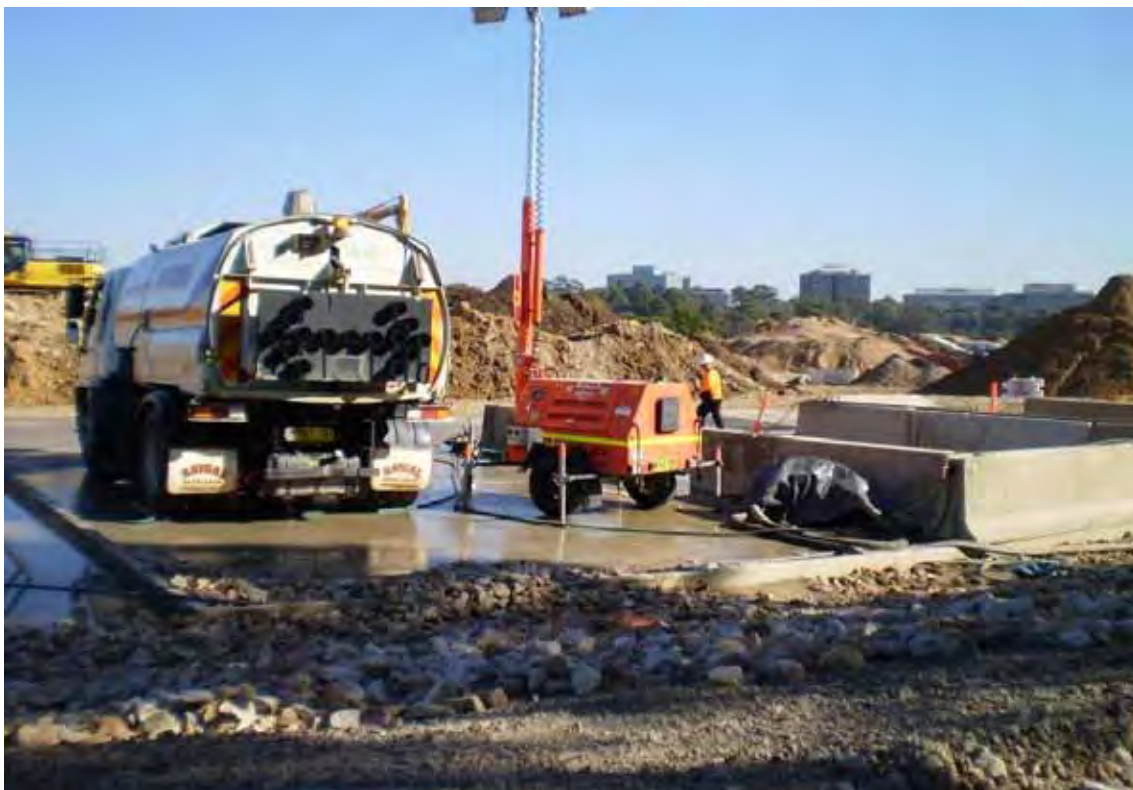
Photo 62 - Vehicle washbay facing north-west
