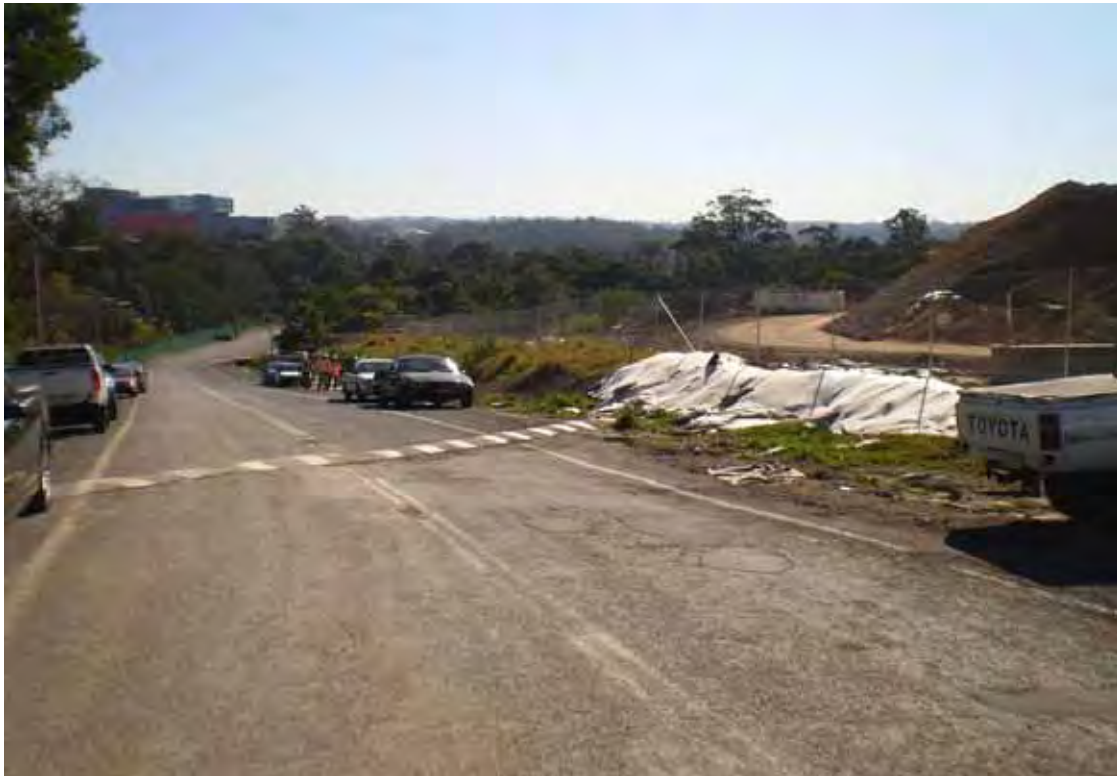
Photo 75 - North along site access road
