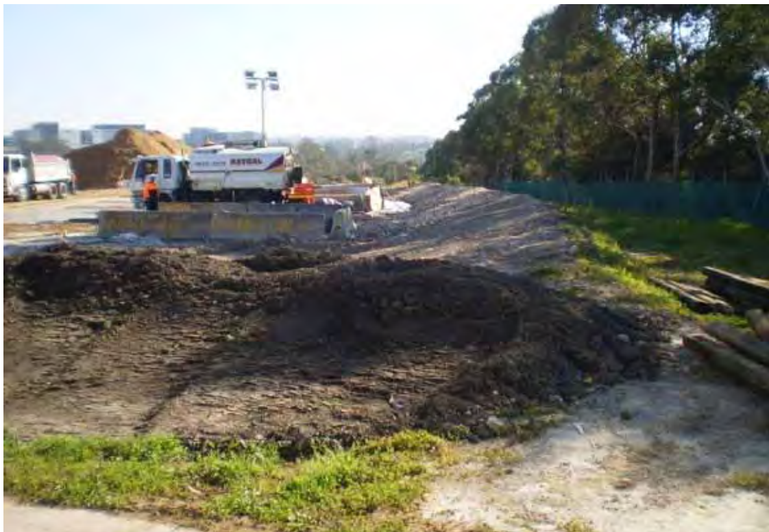
Photo 60 - Bunded wash bay area near eastern boundary to the north of M2 access driveway
