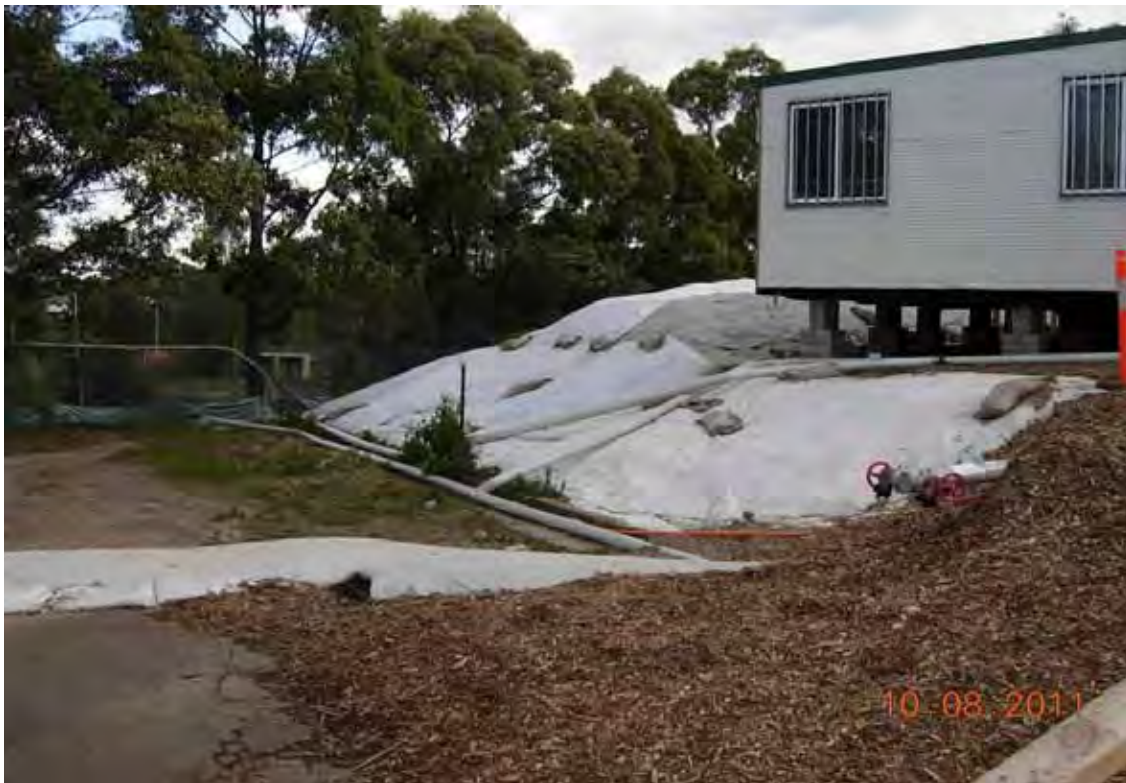
Photo 30 - South western corner of Leighton's sheds facing south-west
