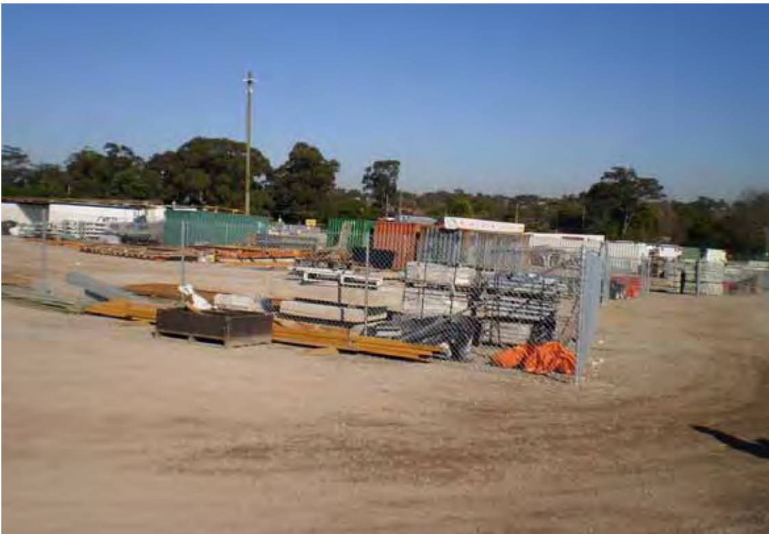
Photo 56 - Storage area within central area of Leighton compound facing south-west
