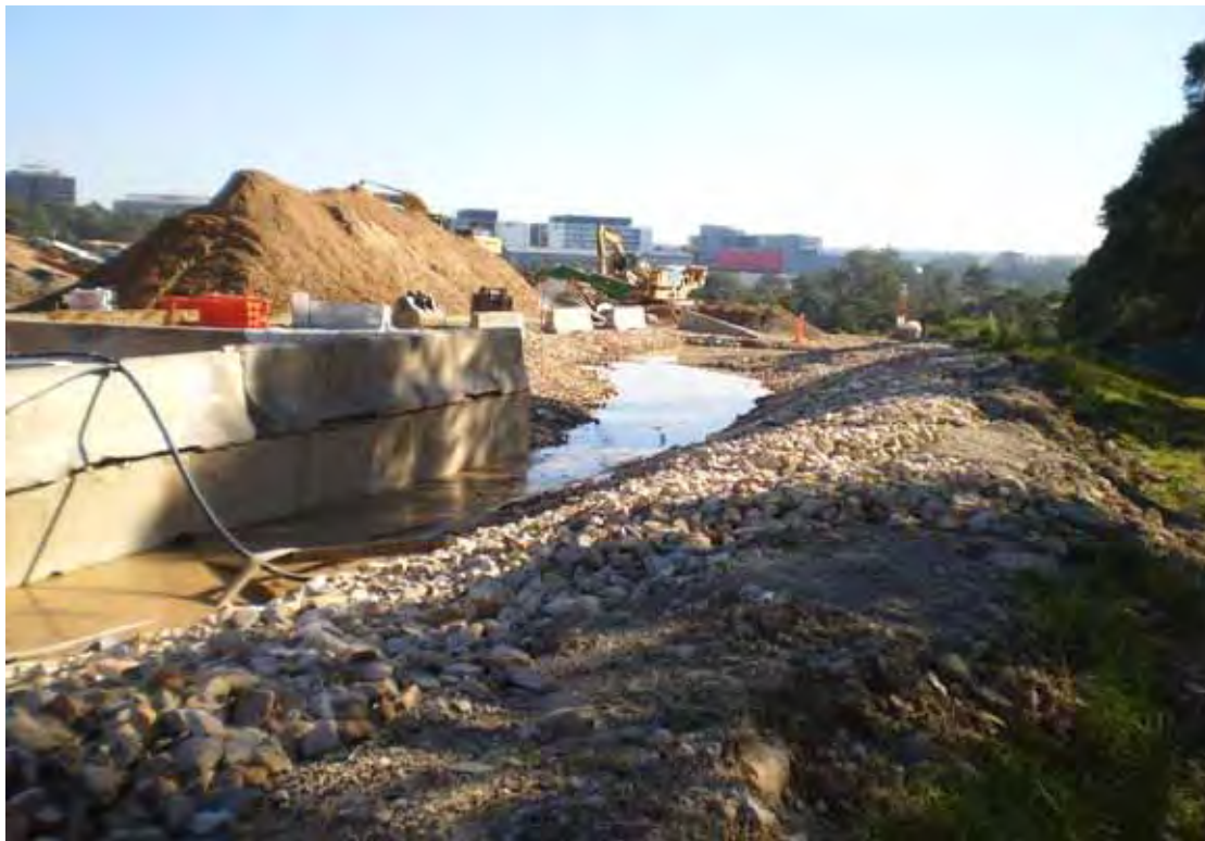
Photo 63 - Drainage of wash bay water towards north of stockpiles
