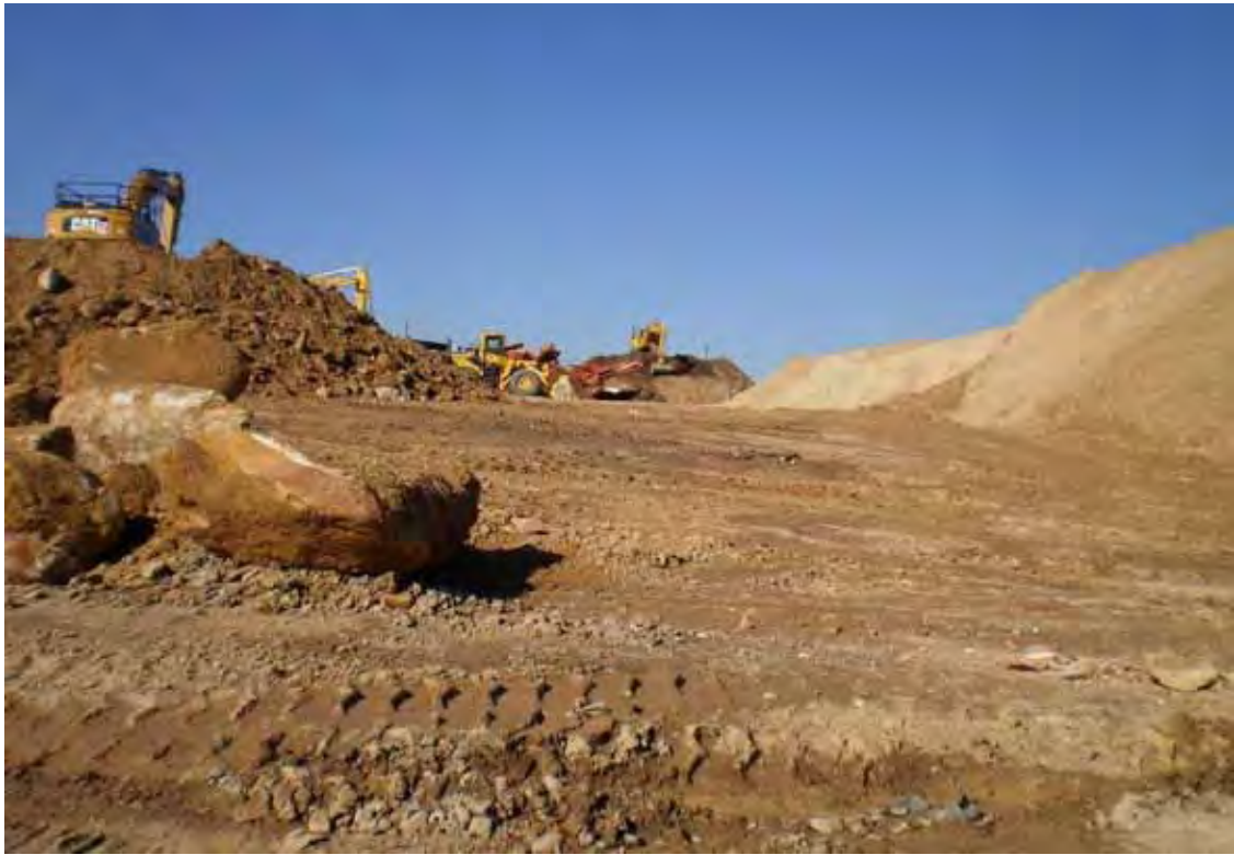
Photo 69 - Stockpiles of material generated from M2 Upgrade works facing south
