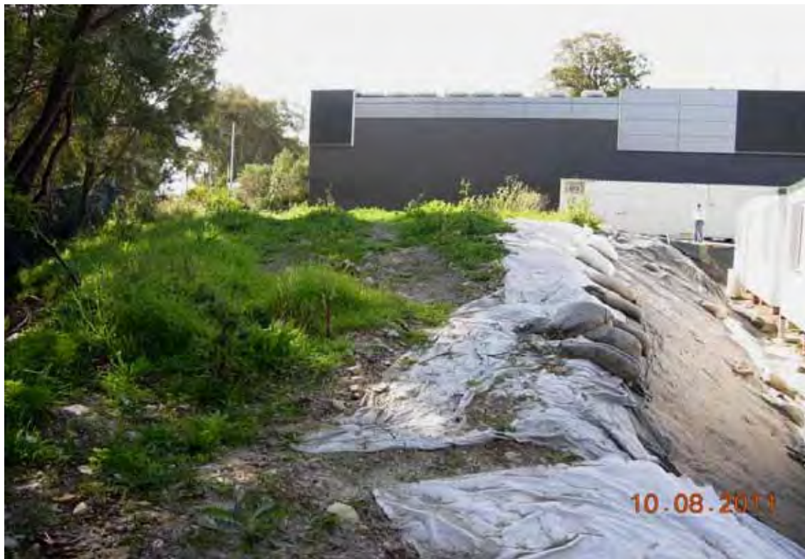
Photo 33 - North-western corner of site facing north
