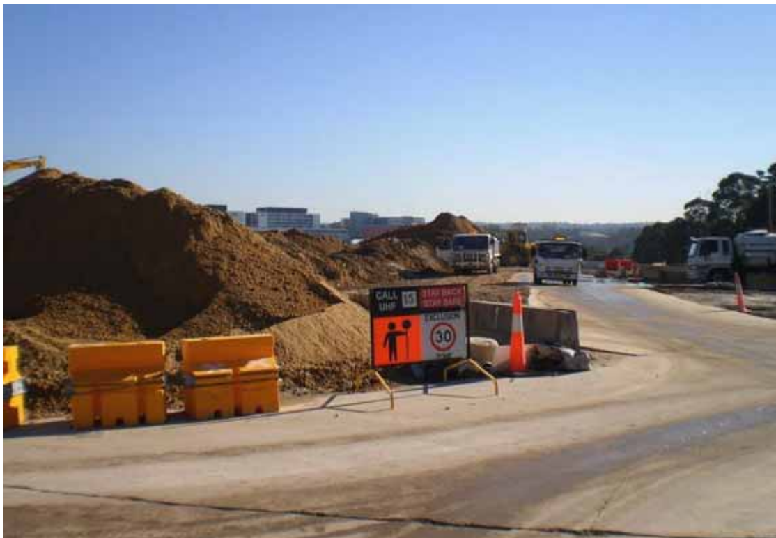
Photo 58 - Vehicle path along eastern side of stockpiles near M2 access driveway
