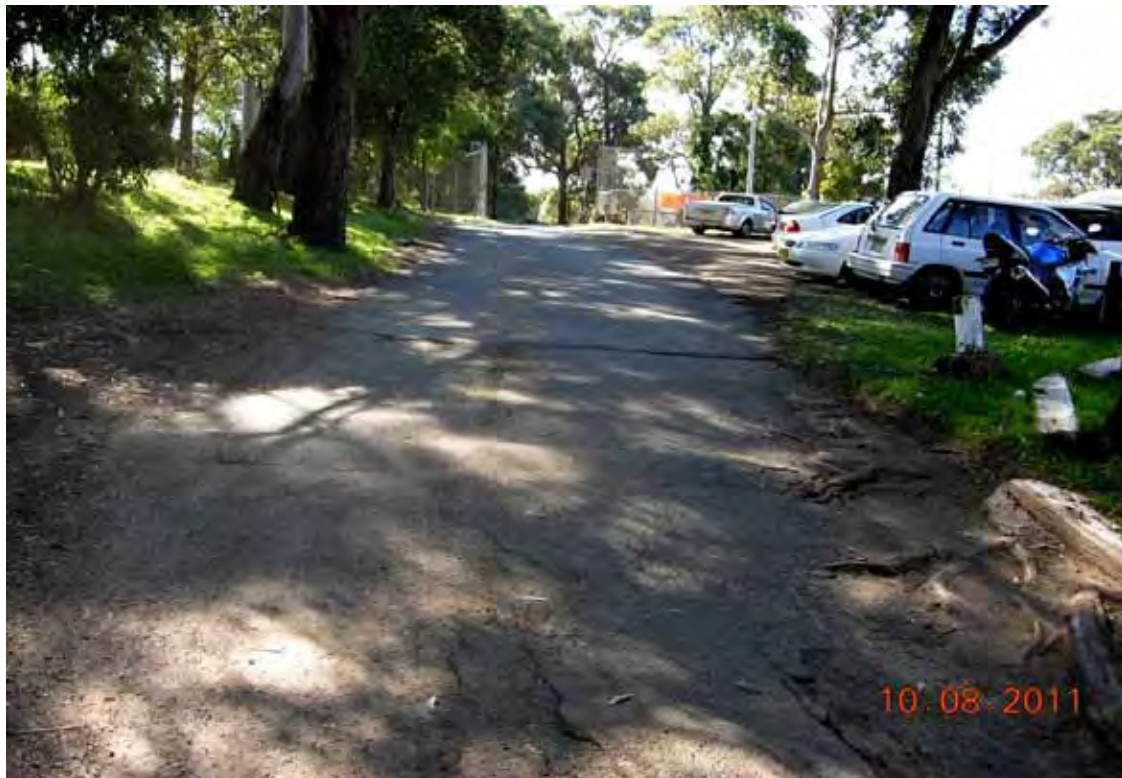
Photo 6 - Drive way facing towards entrance off Epping Road
