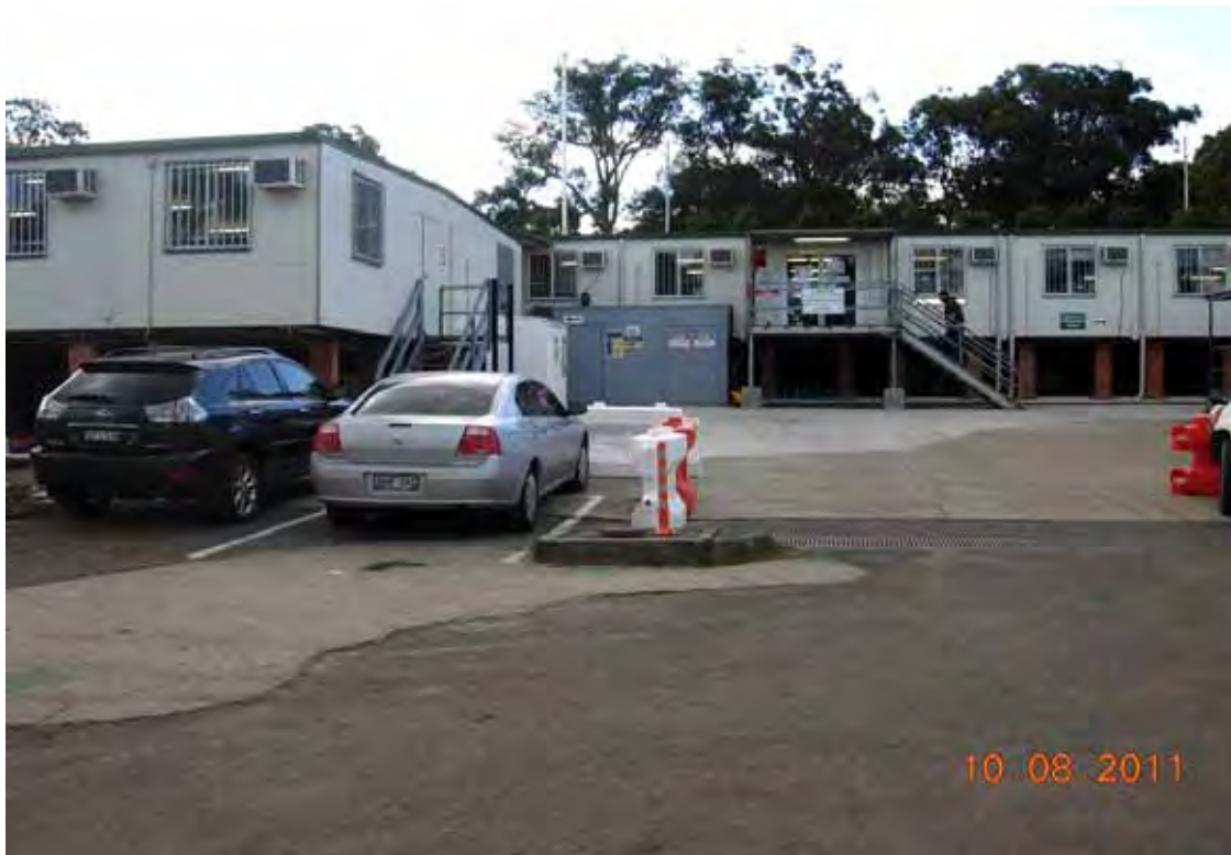
Photo 31 - Within Leighton office shed area facing north
