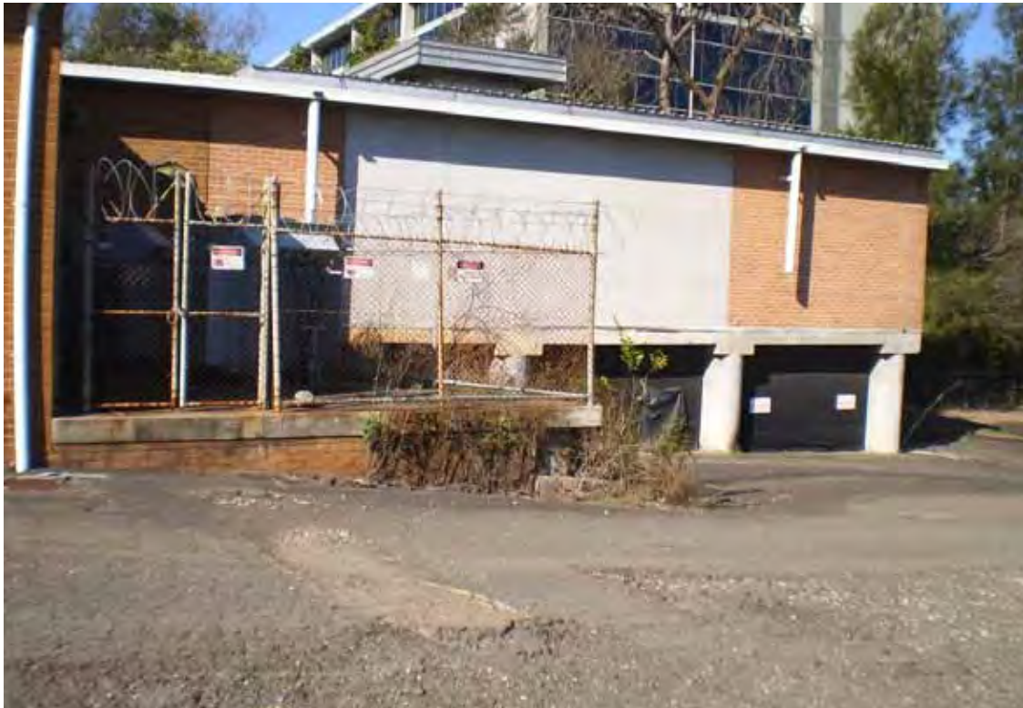
Photo 37 - Substation within former Global TV garage
