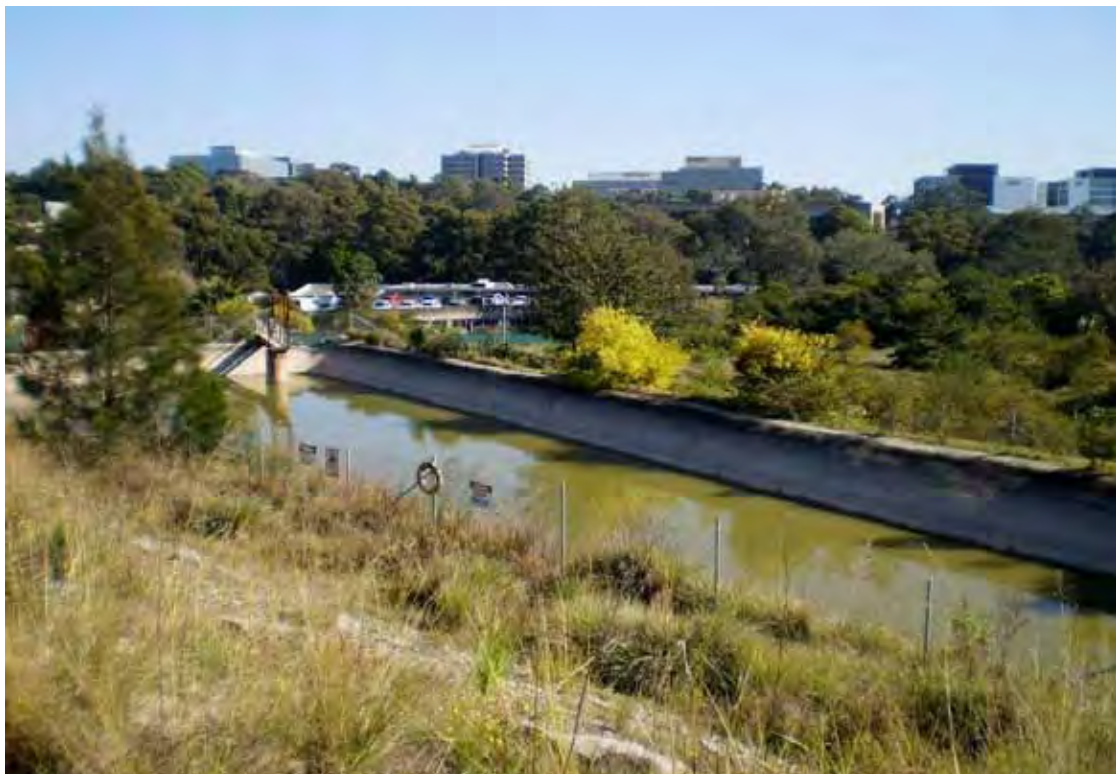
Photo 68 - Detention basin between compound stockpile area and bushland area of site facing north-west
