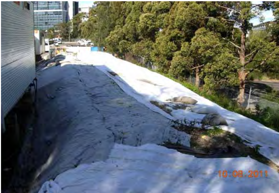
Photo 32 - Southern embankment along Leighton sheds facing east
