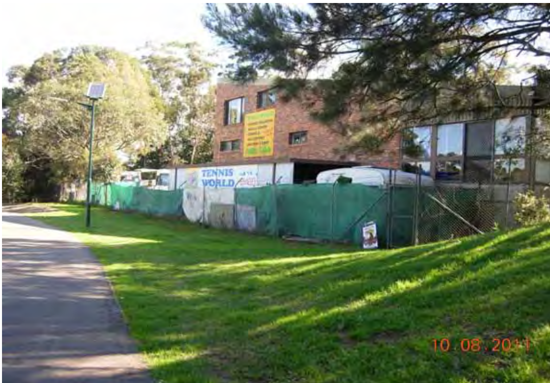
Photo 10 - Facing south-west along south-eastern boundary from within neighbouring Blenheim Park
