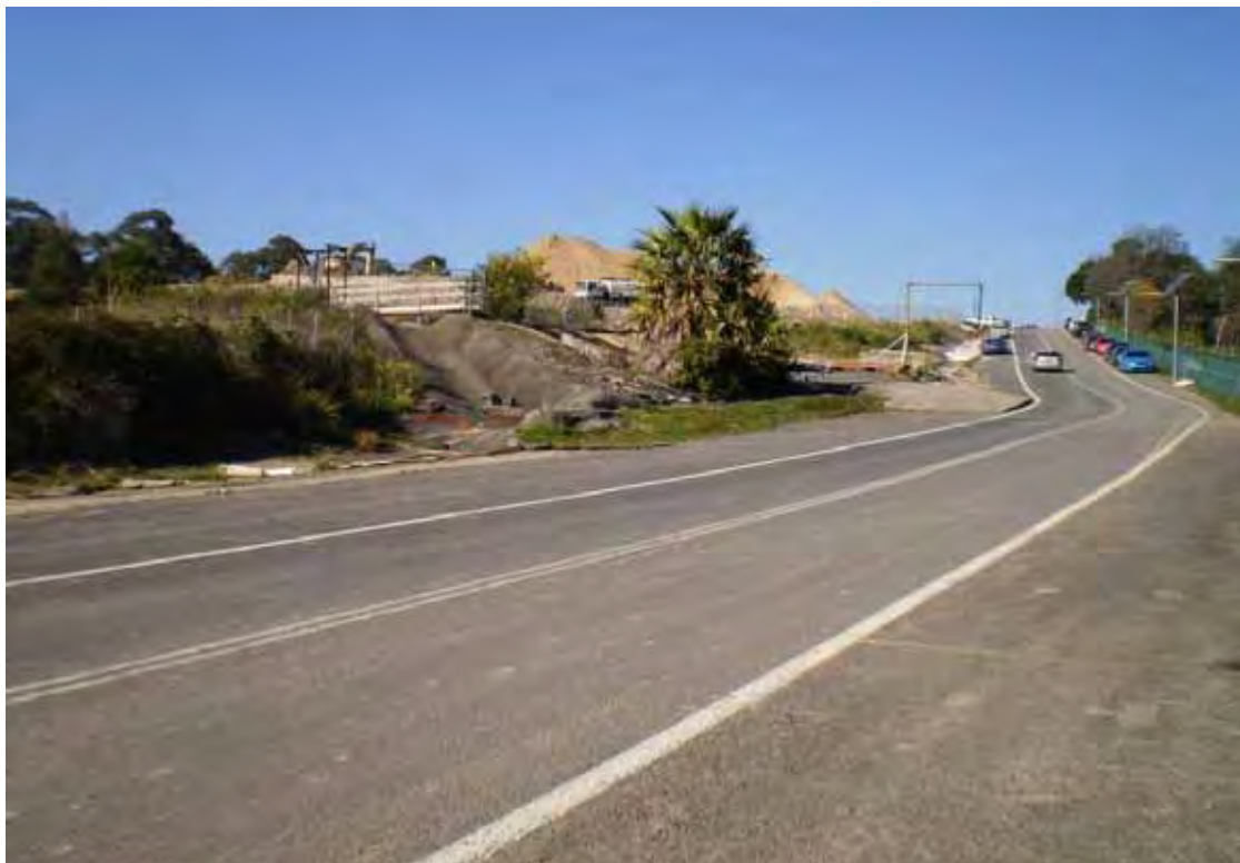
Photo 76 - South along site access road with detention basin and stockpiles located in centre of image
