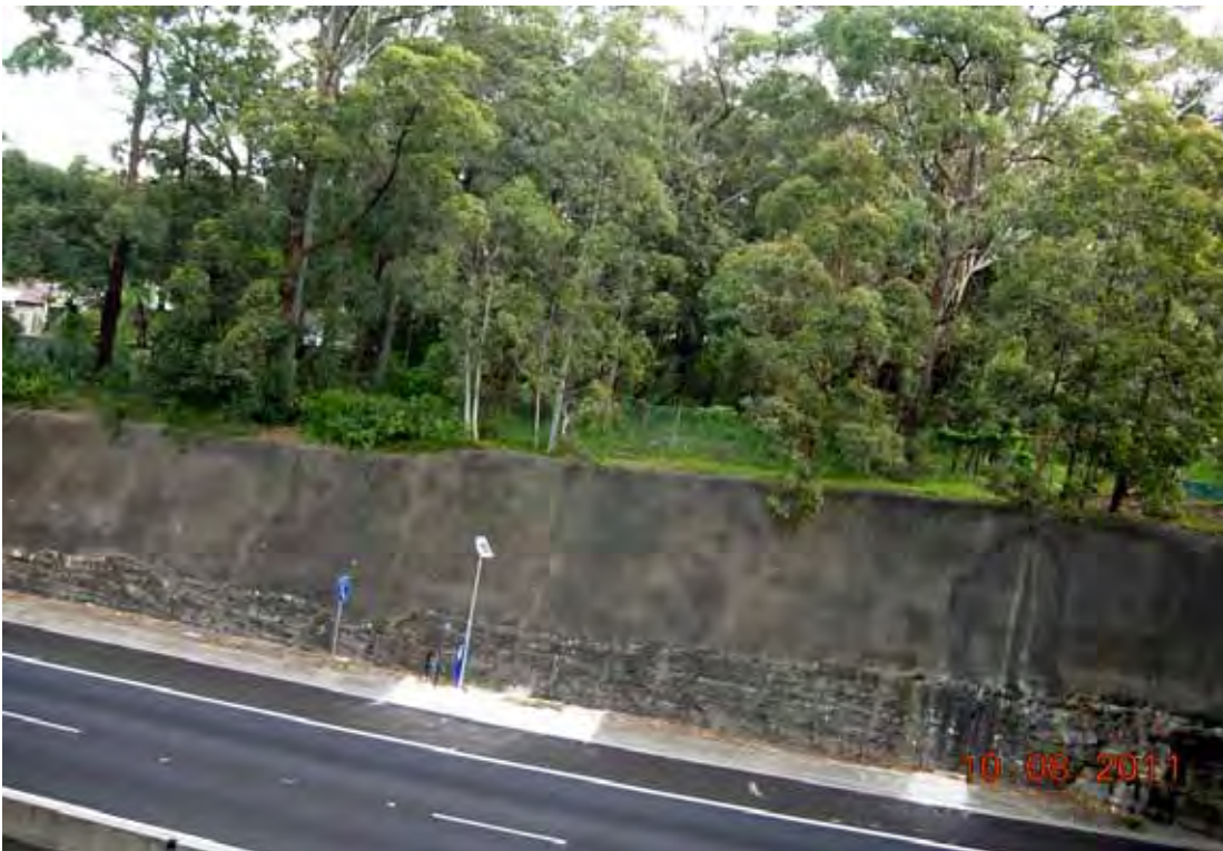
Photo 20 - Eastern boundary of site at M2 Motorway facing south-west
