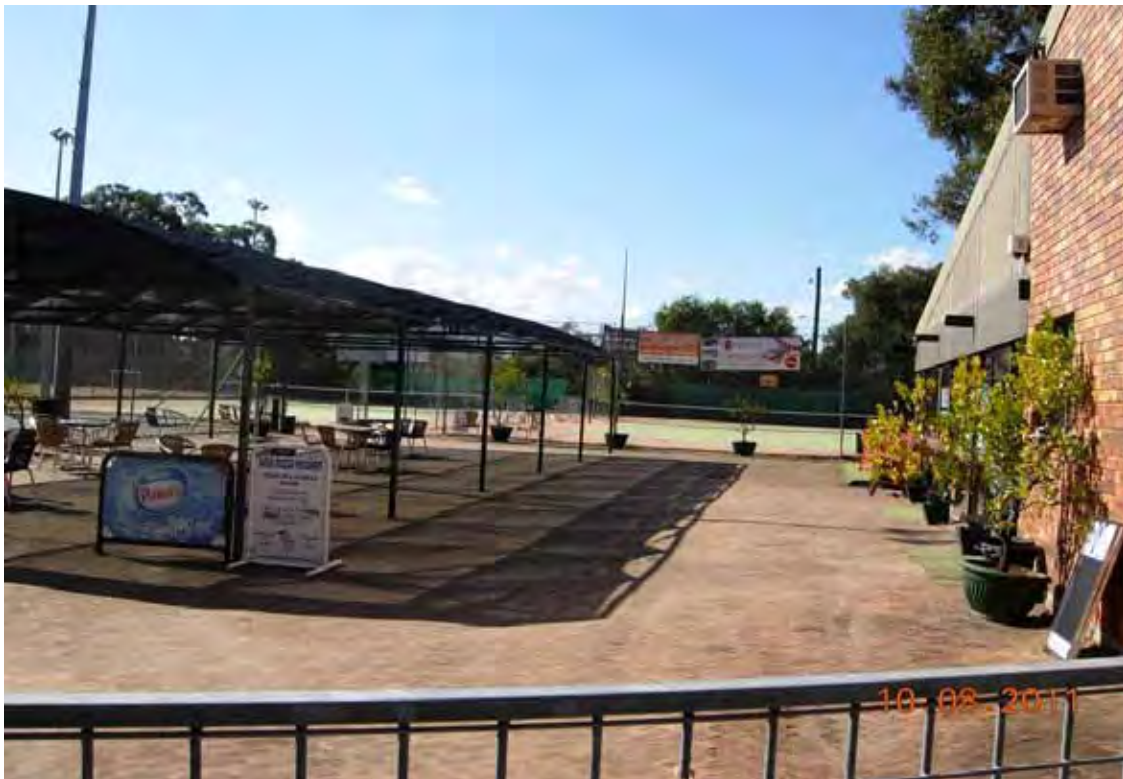
Photo 8 - Club house/shop and courtyard area facing north-east towards Epping Road
