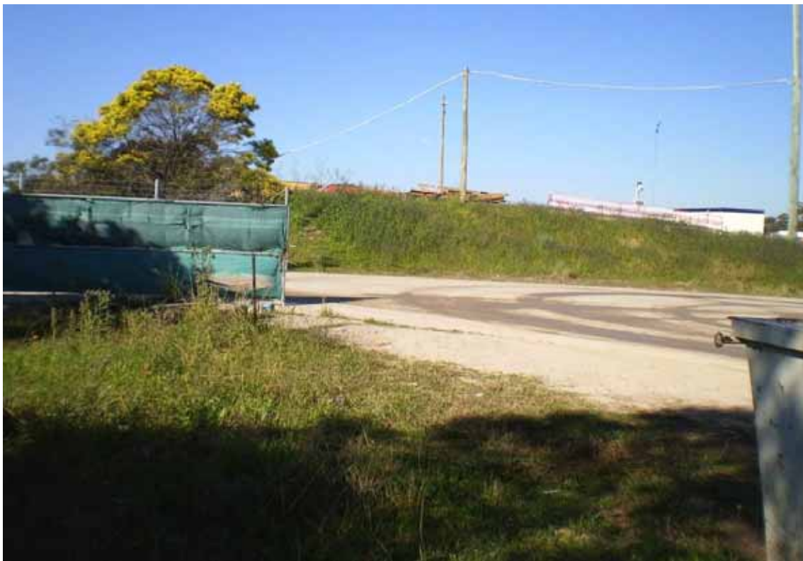
Photo 61 - Embankment at M2 access driveway facing south
