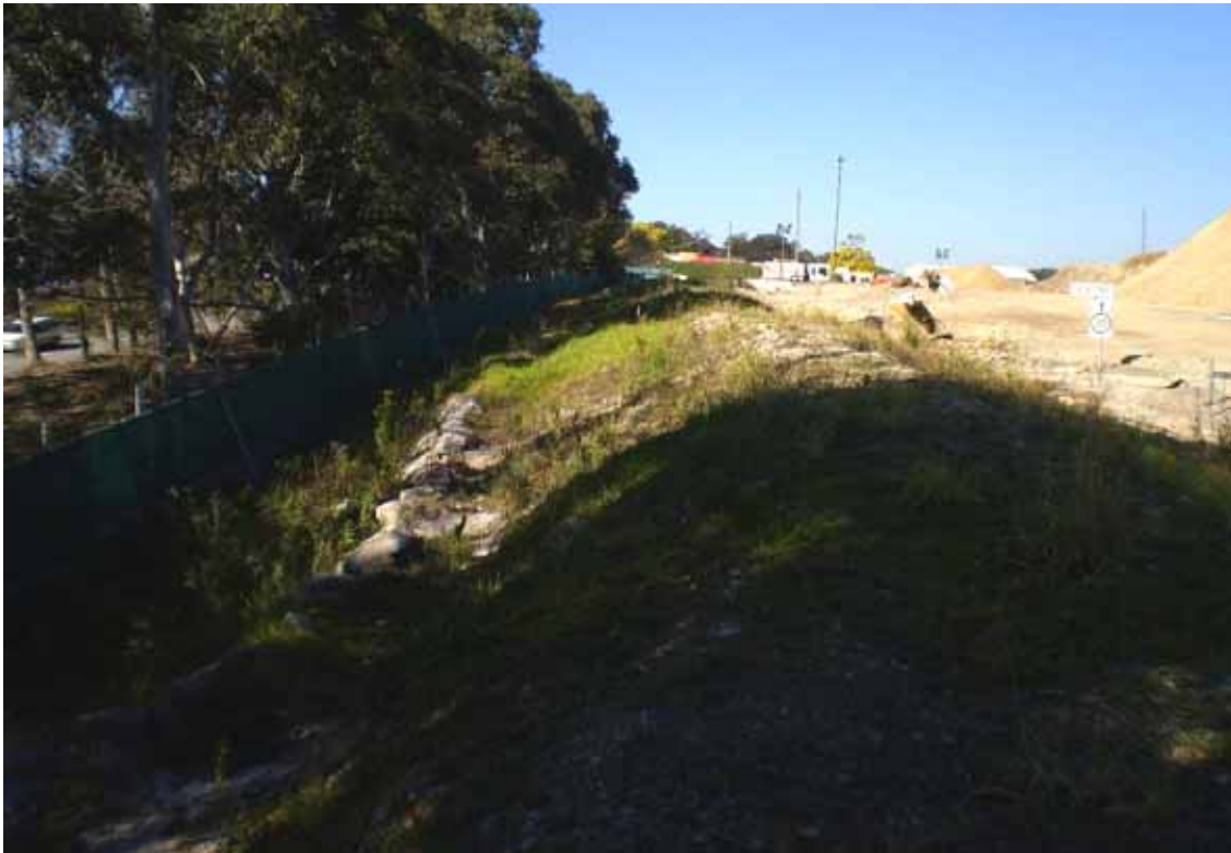
Photo 65 - Embankment along eastern boundary facing south
