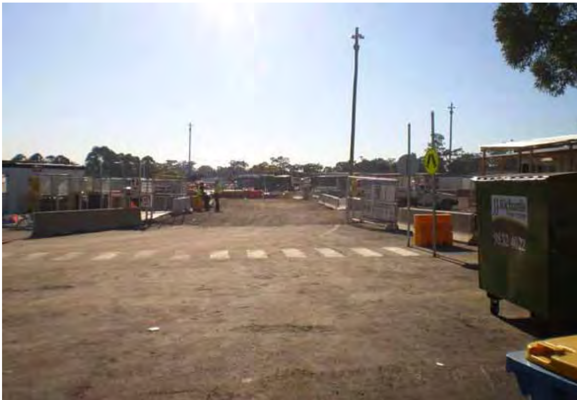
Photo 48 - Facing north-east with site office sheds to right of image
