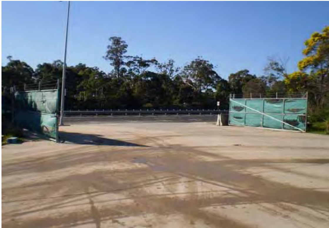
Photo 59 - Vehicle access into site from M2 facing east onto M2
