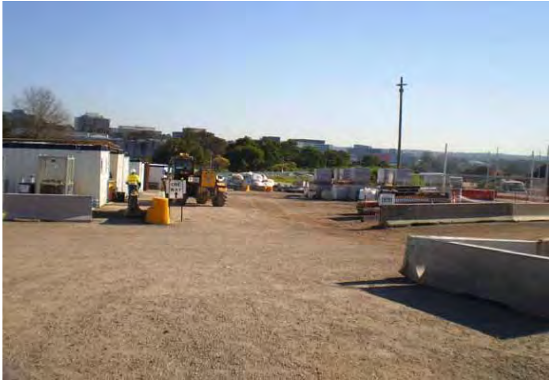
Photo 49 - Facing north-west from in front of site office shed area
