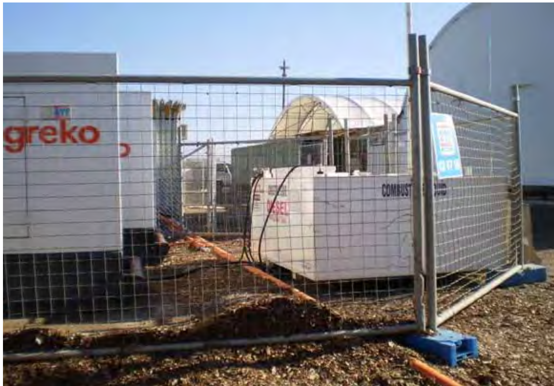
Photo 51 - Generator and deisel tank for refueling located near southern site boundary near site office sheds
