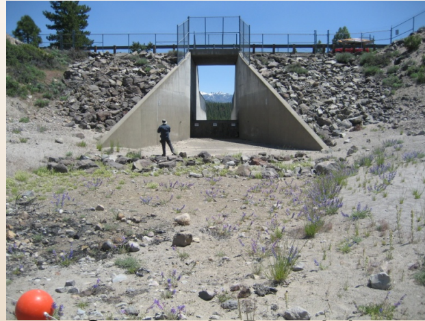
Stampede Dam Inlet Control Structure
