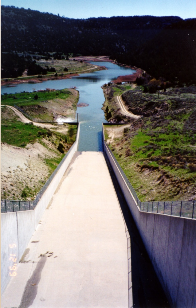
Glendo Dam Chute Walls
