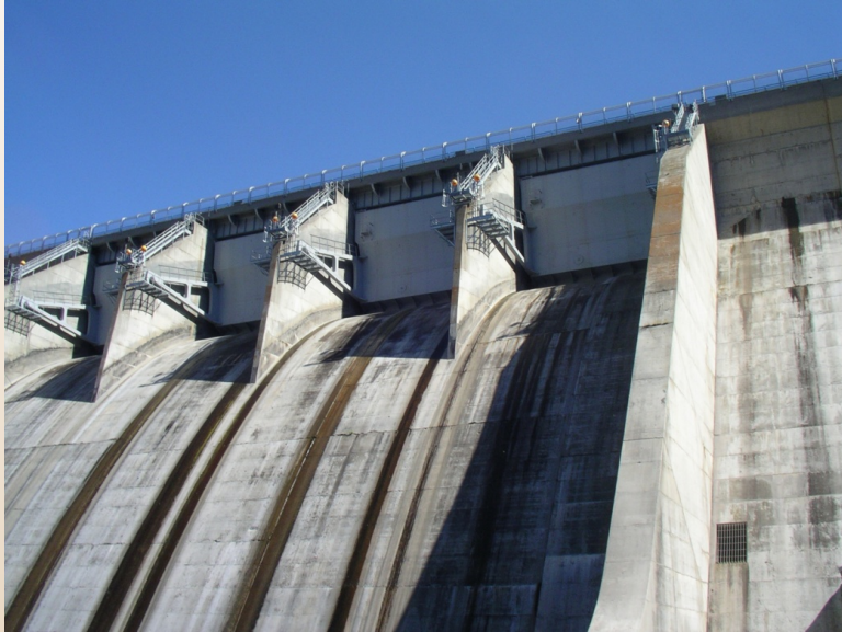
Spillway Gate Piers
