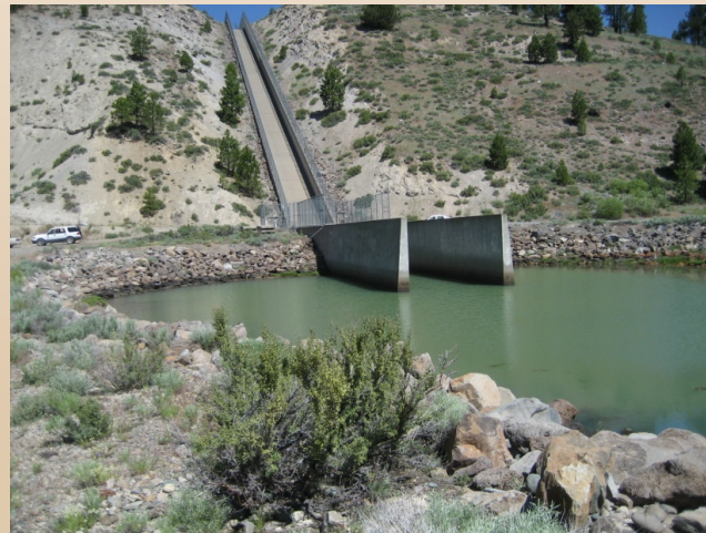
Stampede Dam Stilling Basin
