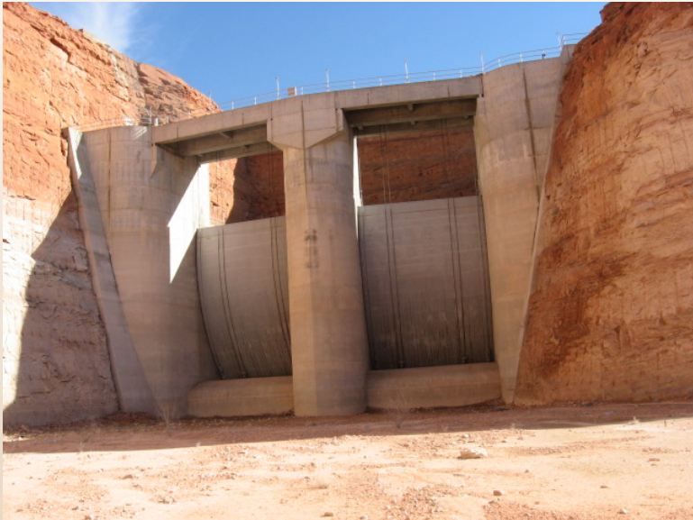
Spillway Gate Piers
