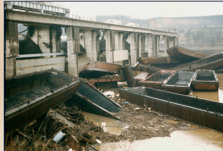
Damage from Barge Impact
