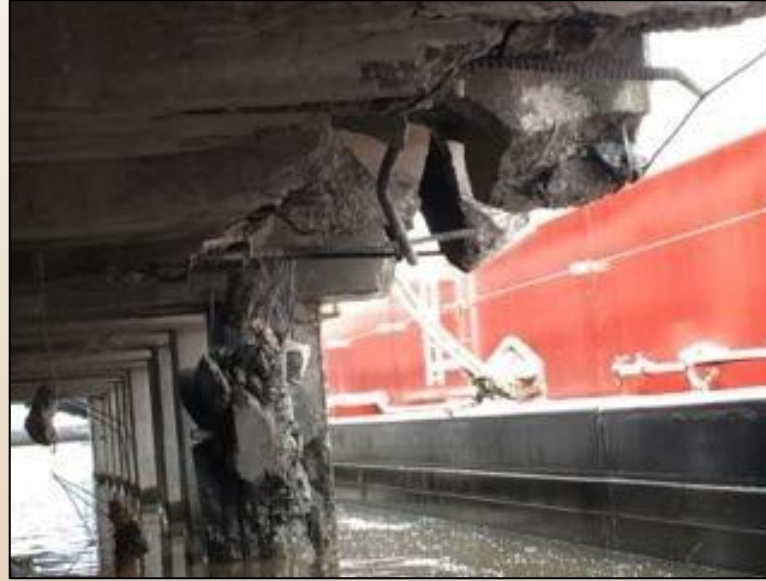
Damage from Barge Impact
