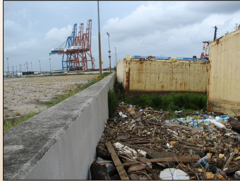
New Orleans Floodwall: 2005 Katrina
