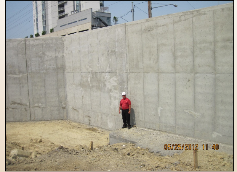
Newport, KY Floodwall
