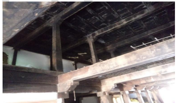
Fig. 10. Wooden Columns and Rafter
