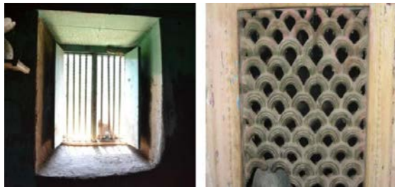
Fig. 5. Small Windows and Jaali on the exterior wall
