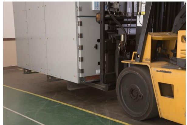
Figure 5: Lifting of switchgear frames with forklift
