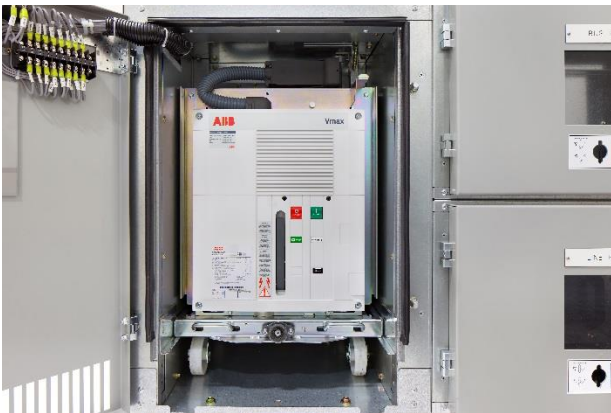
Figure 22: Vmax/A in test position
