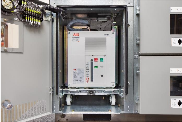
Figure 21: Vmax/A in disconnect position
