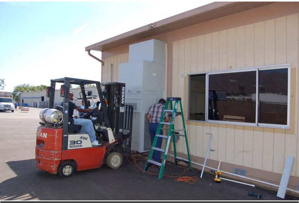
Installation of CH4S1-A
