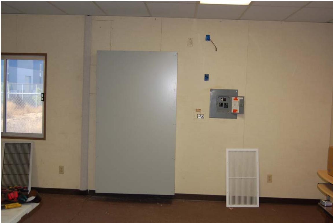
Interior with Return Air Acoustical Plenum installed.
