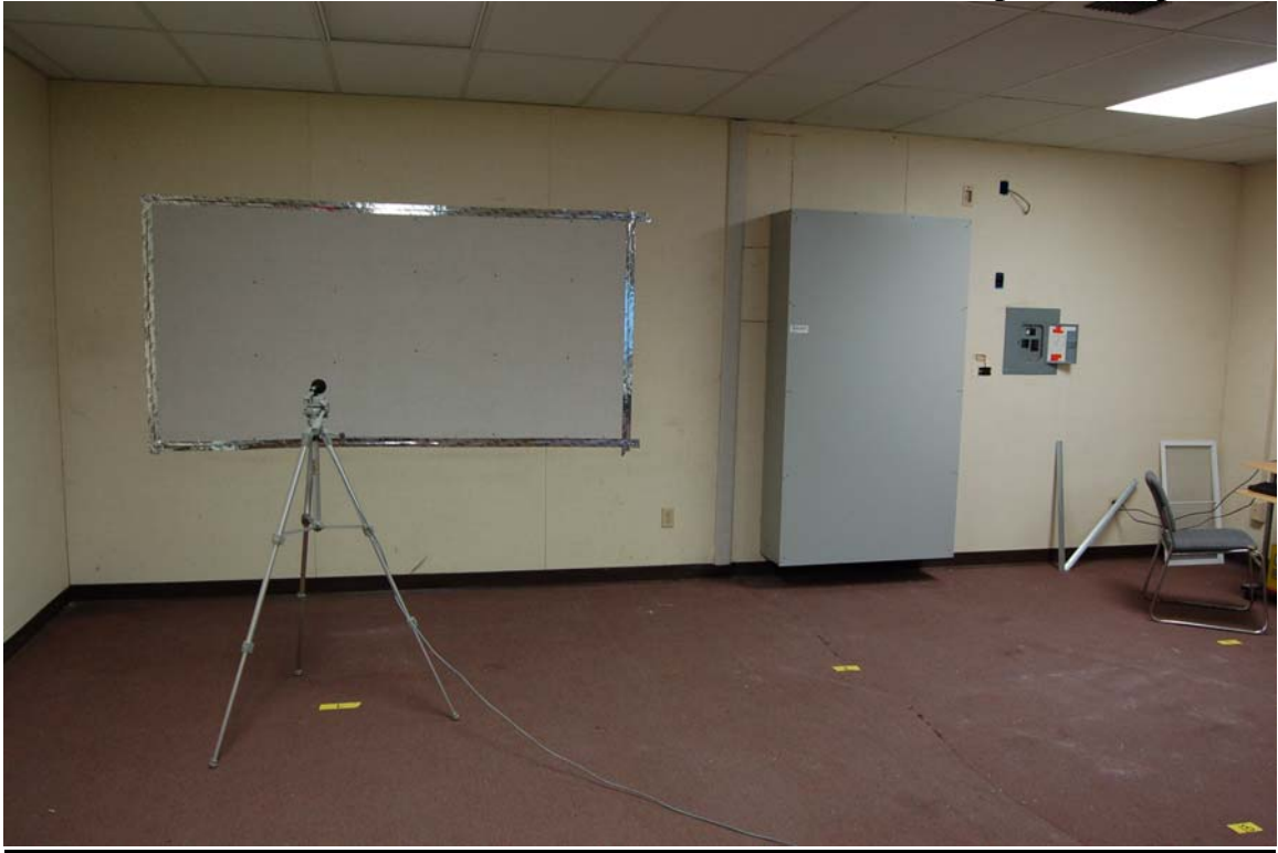
Interior with end wall window removed and return air acoustical plenum in place.
