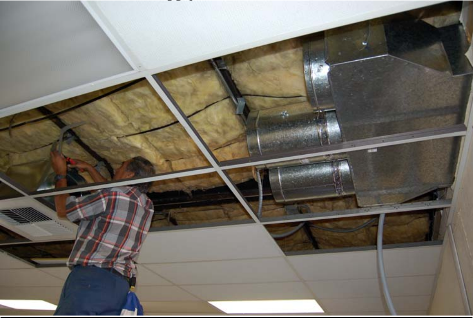
Installation of 3 outlet supply ducts
