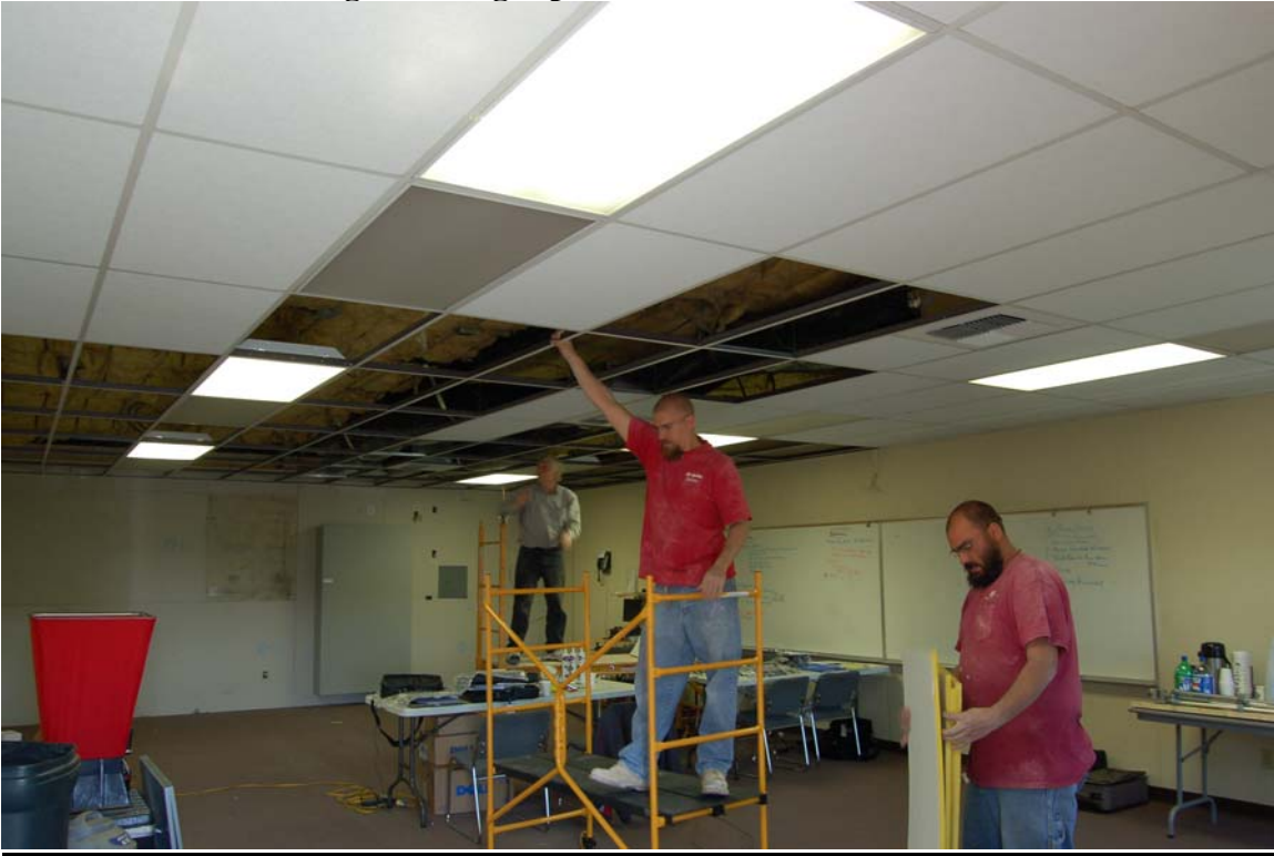
Interior with the ceiling tile being replaced.
