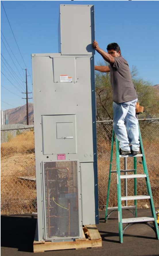
CH4S1-A with Top Plenum being installed
