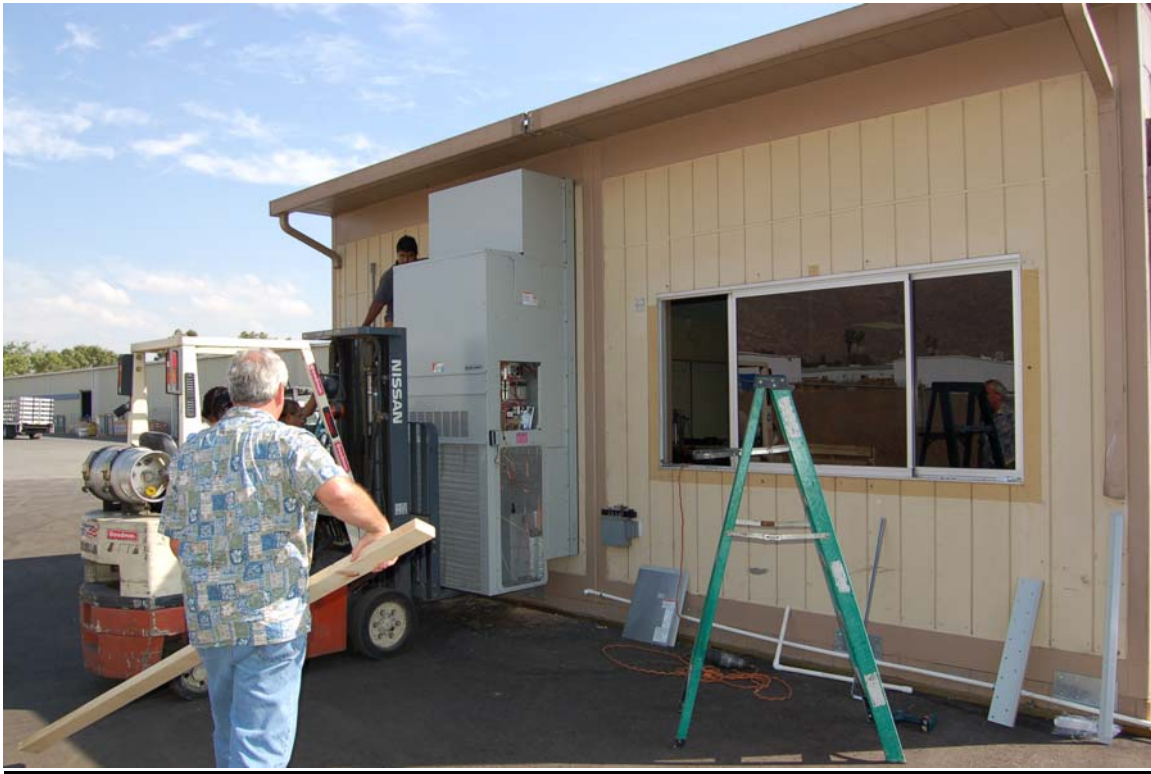
Installation of CH4S1-A
