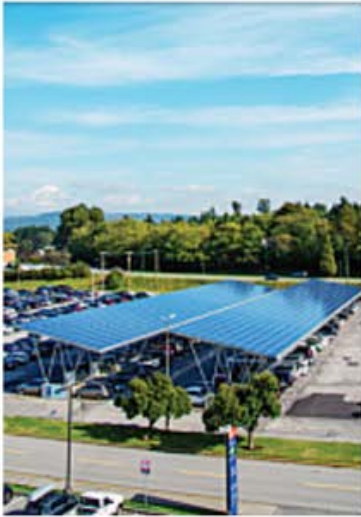
Microgrid and Energy Management Systems
