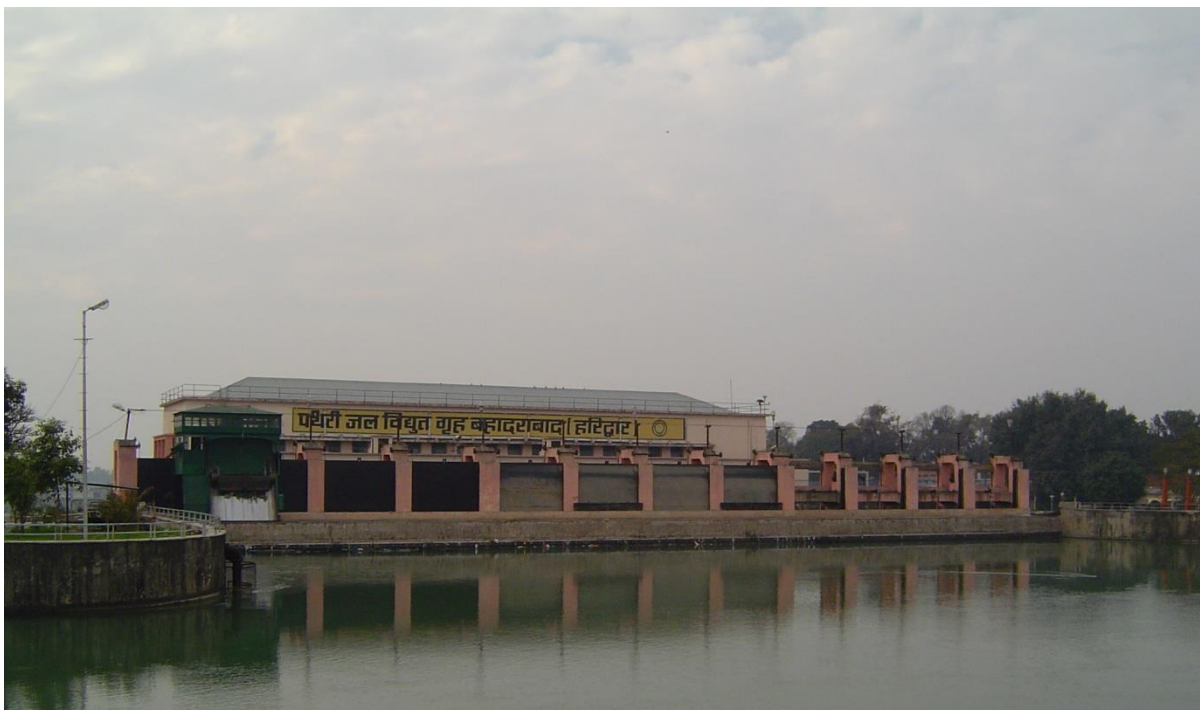
Figure 2: Pathri Small Hydro Power Plant
