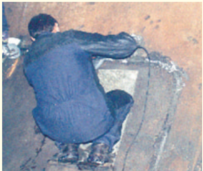
Figure 3. Grinding of the joint on the inside of the kiln.
