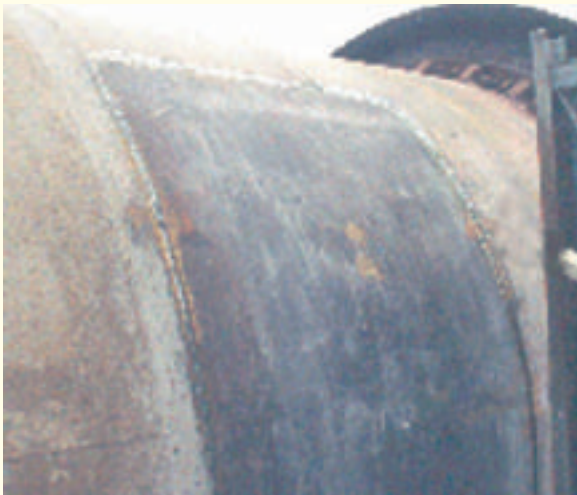
Figure 2. The replacement plate after welding.
