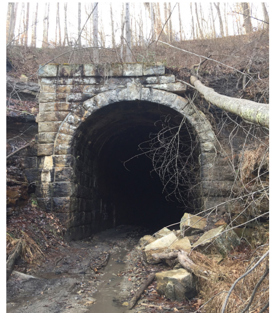
East portal of the Kingsville Tunnel. Photo by Janis Bland
