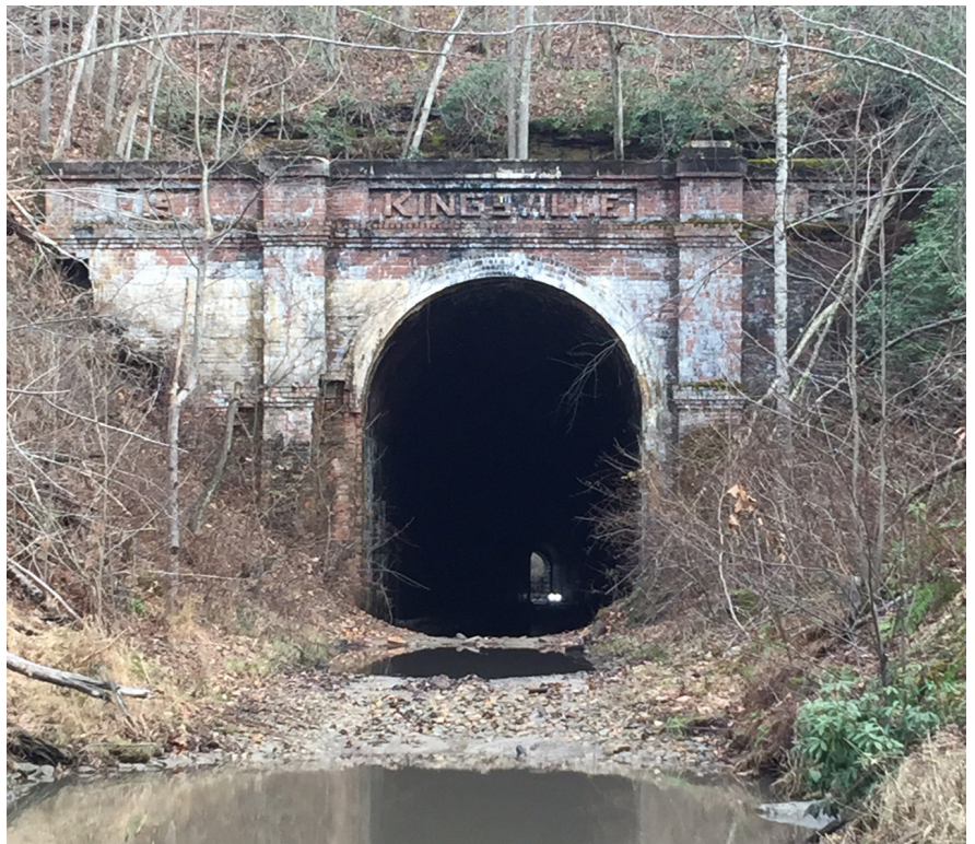
West portal of the Kingsville Tunnel, with 1924 brick facade.
