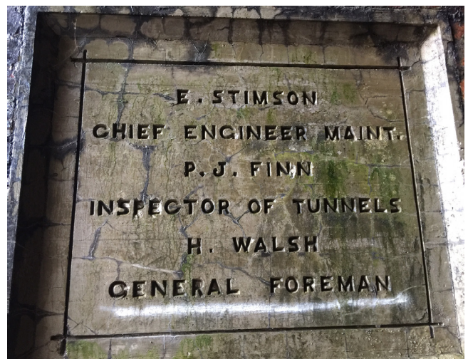
Builders' Plaque at the east portal of Kingsville Tunnel. Photo by Janis Bland (Continued on Page 6)
