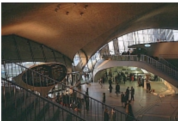
Interior view of main level of terminal
