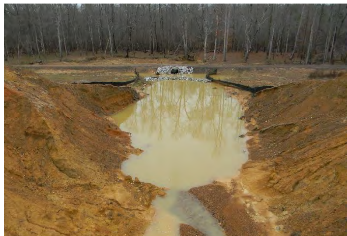
View of Dam Failure Looking Downstream
