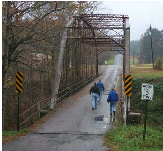
Courtesy of the Alabama Department of Transportation
