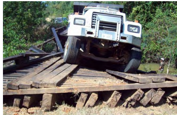
Posted Bridge Crossed by Dump Truck Courtesy of the Alabama Department of Transportation:
