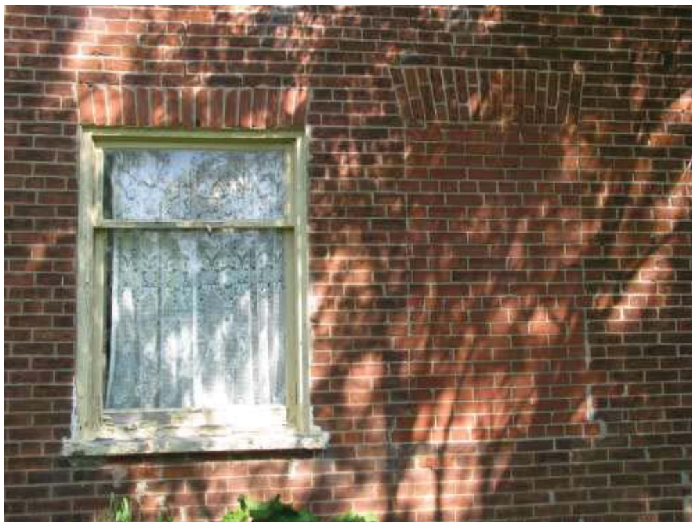
Plate 8: Detail of windows showing one bricked over
