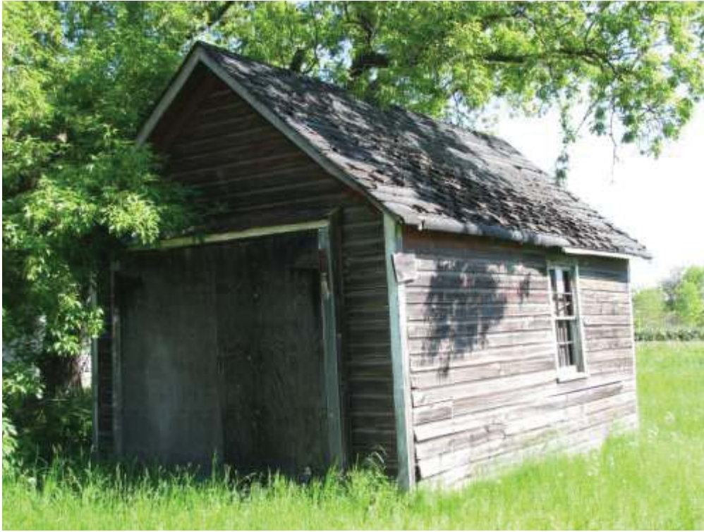
Plate 17: Wood frame garage
