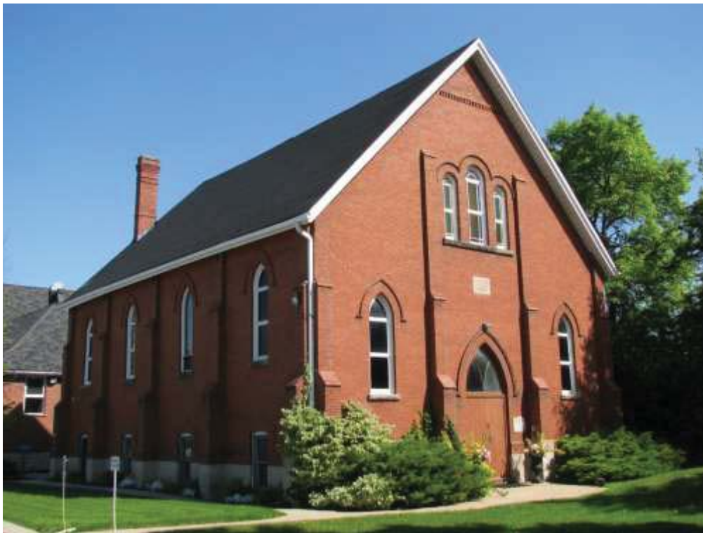
Plate 3: 1898 Munn's Methodist Church, now Munn's United Church, facing northeast
