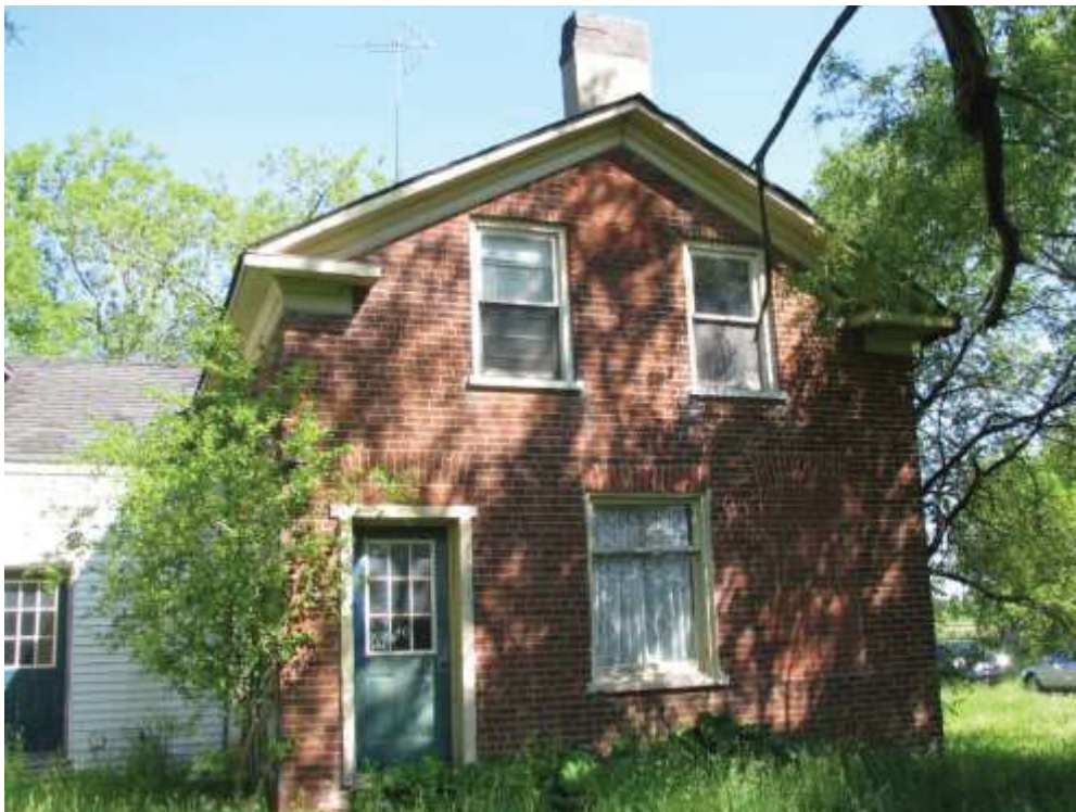
Plate 16: Detail of cornice returns and cambered window heads
