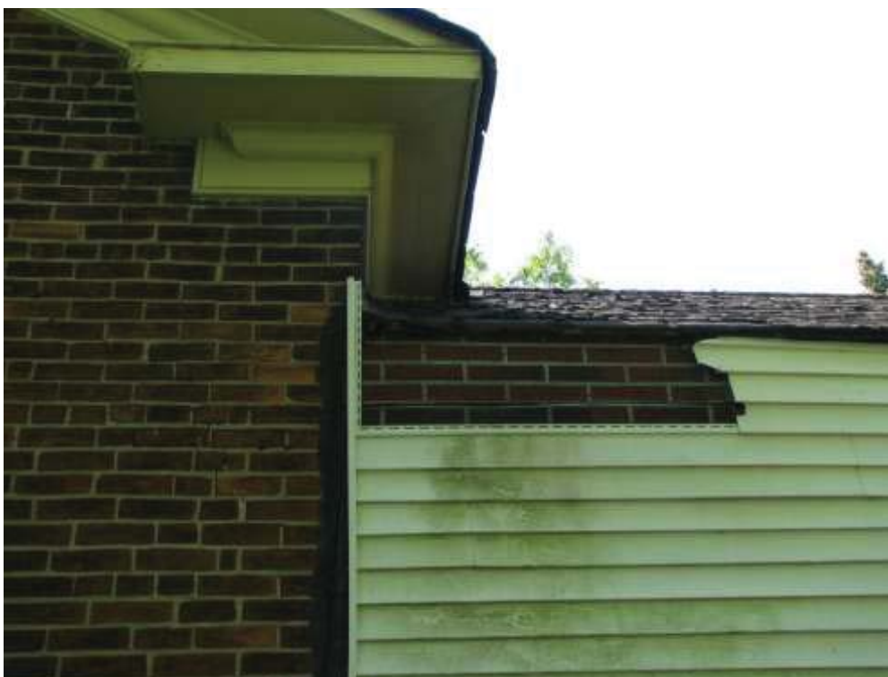
Plate 11: Detail of vinyl siding over imitation brick siding
