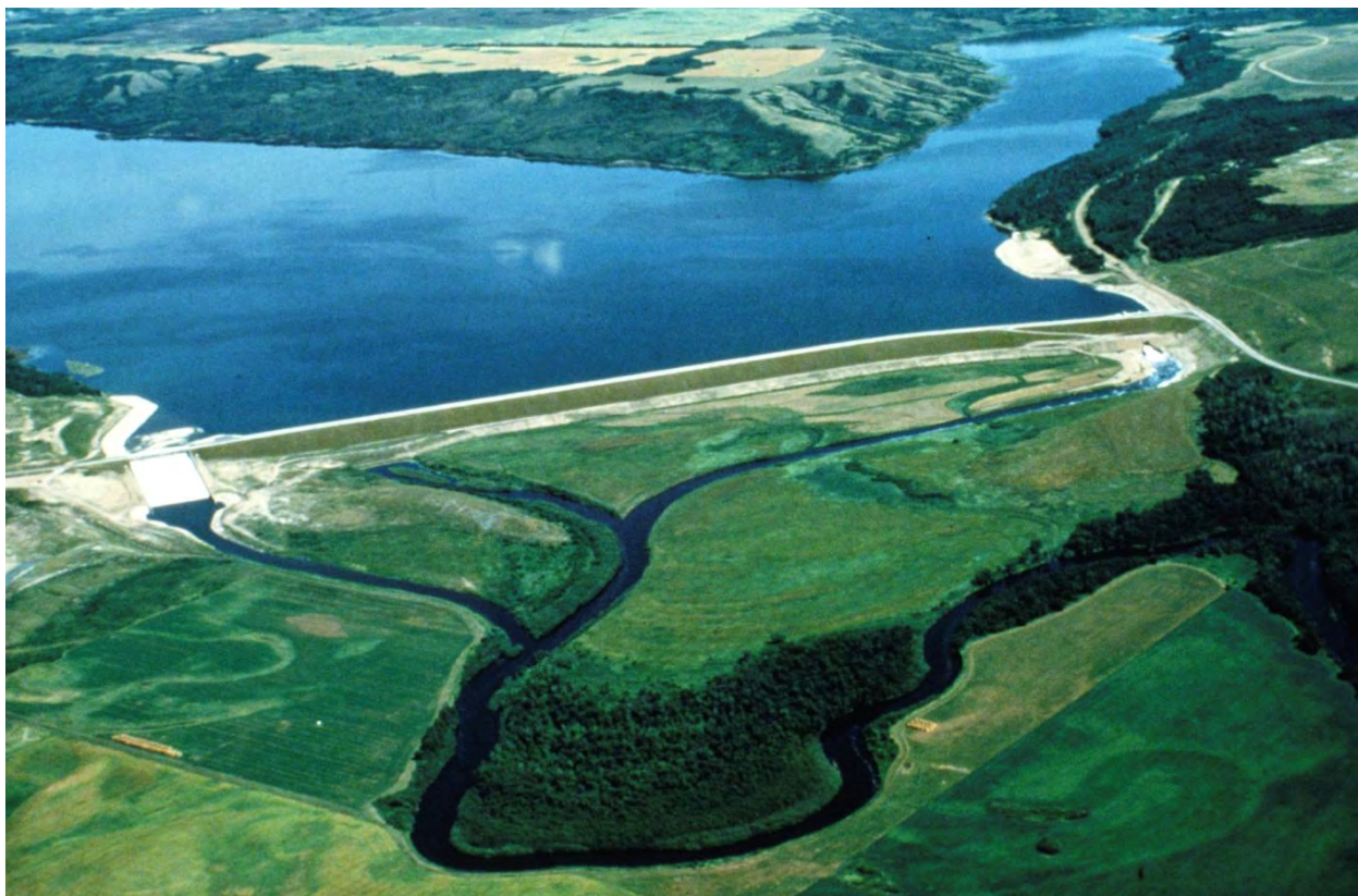
Figure 1: An aerial view of Shellmouth Dam and Reservoir (Lake of the Prairies) looking upstream. Upper right is the Shell River. The outlet is on the right hand side of the photo and the spillway is on the left hand side of the photo.
