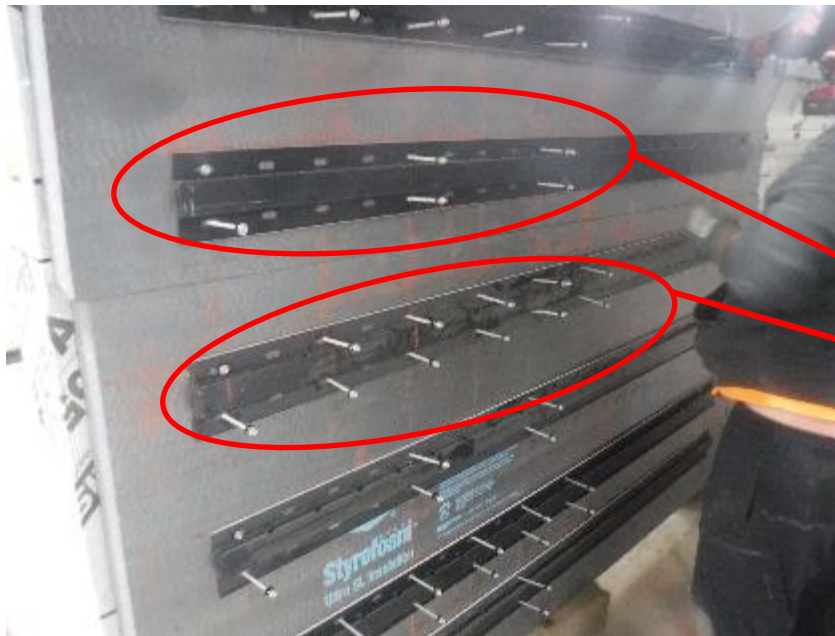
Photograph No. 10 Knight Wall Installation Fastener placement. 16" O.C. 8" O.C
