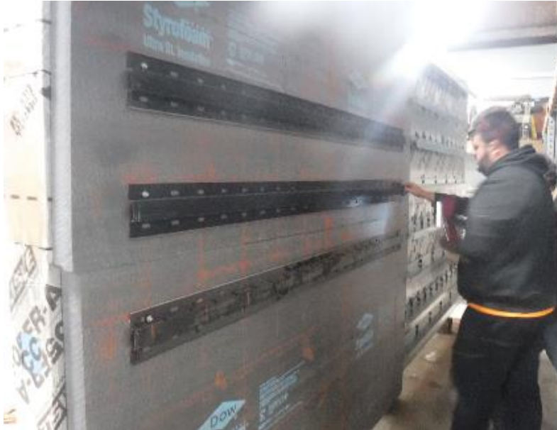
Photograph No. 9 Knight Wall Installation HCl-GIRTs being installed
