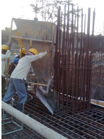
Figure 14: Concrete being poured in the column formwork and the Reinforcement
