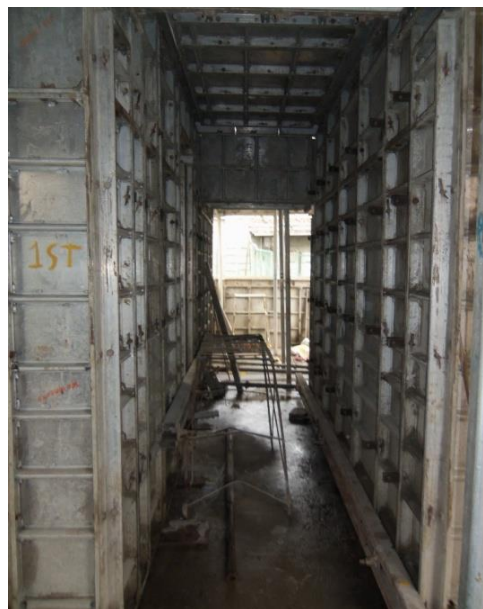
Figure 4: Aluminium Formwork
