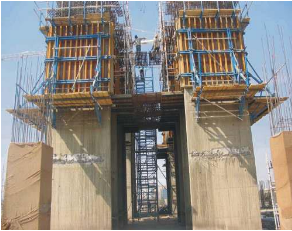
Figure 10: Climbing Formwork
