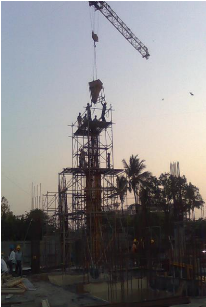
Figure 13: Concrete being poured in the column formwork and the Reinforcement
