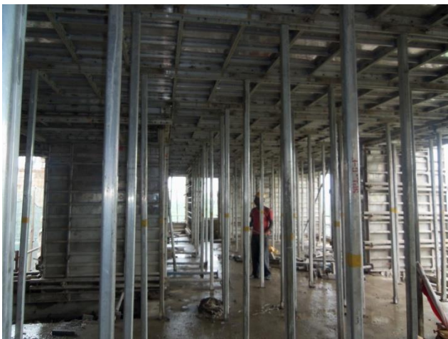
Figure 19: Setup of formwork
