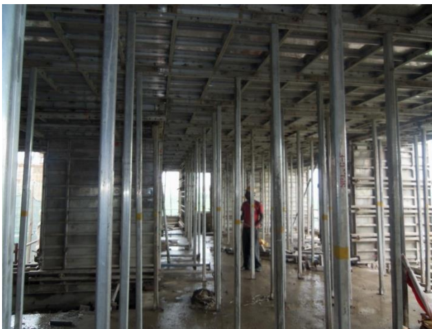
Figure 3: Aluminium Formwork
