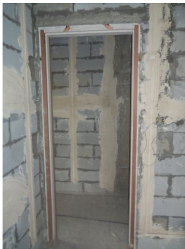
Figure 24: Door Frame being fixed
