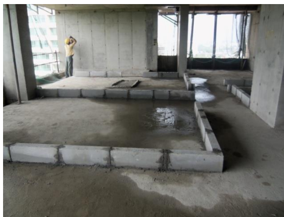
Figure 20: Laying of Blockwork
