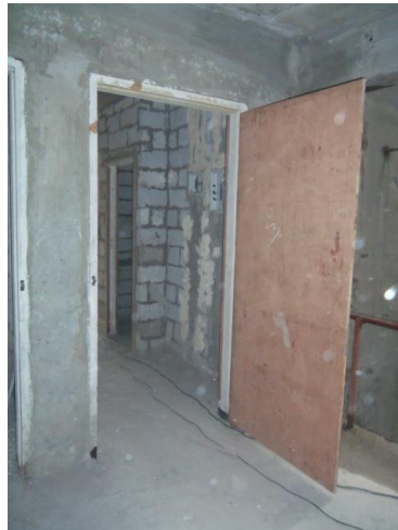
Figure 23: Door attached to the frame
