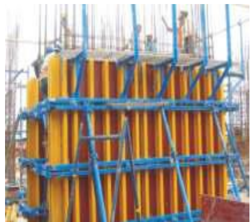
Figure 12: Climbing formwork
