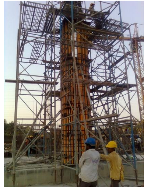
Figure 5: Circular formwork for the column
