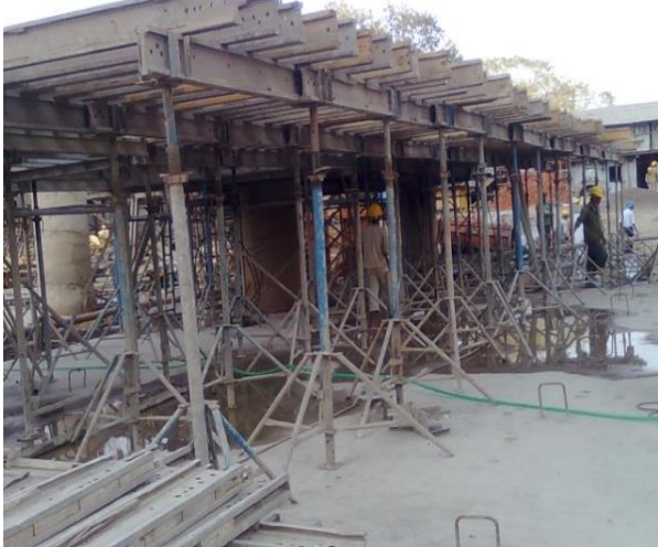
Figure 6: H-Beams laid for first floor slab
