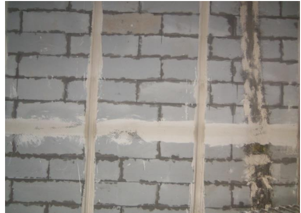
Figure 21: Mesh fixed at junctions
