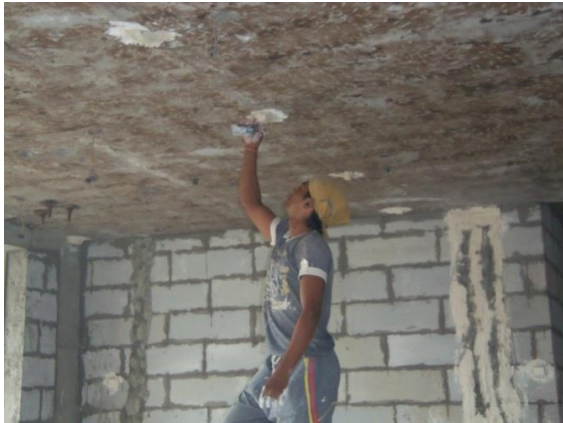
Figure 22: RCC being chiselled
