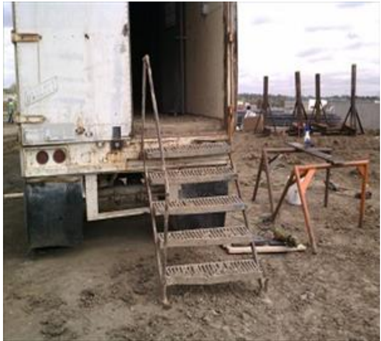
These stairs need to be repaired or replaced!
