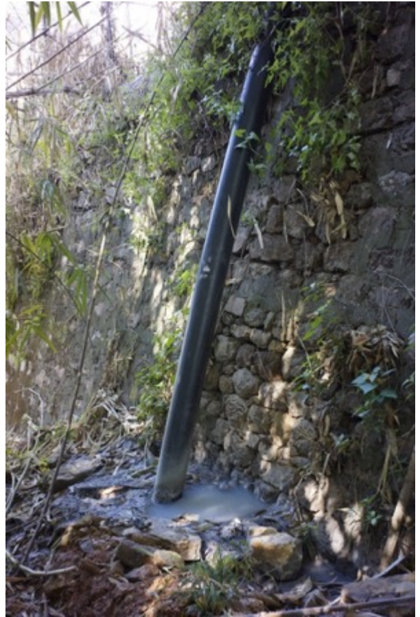
Disposal of grey water used by washing room
