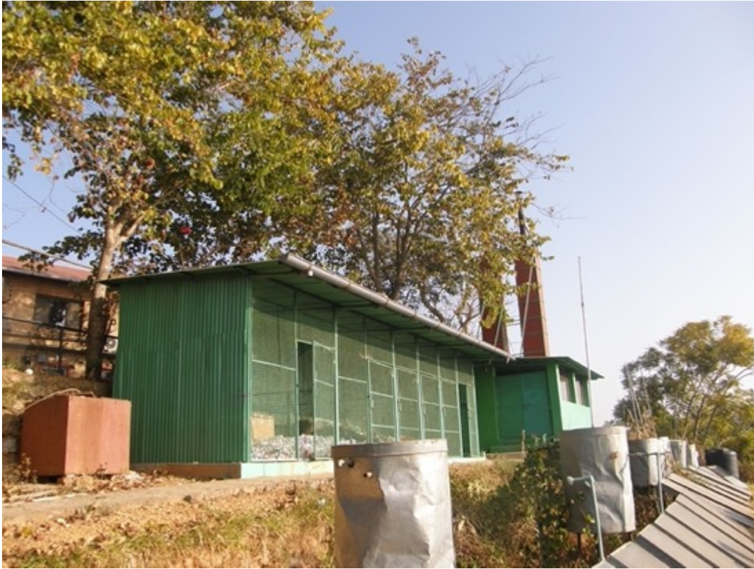
Waste separation building; at the back incinerator
