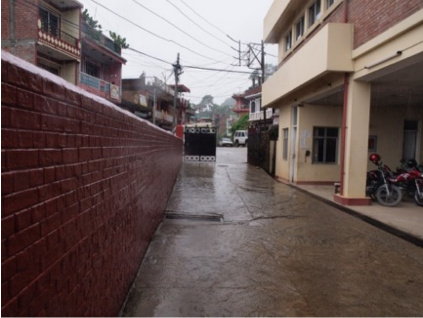
During rains, rainwater from pavement mixes with black waste water
