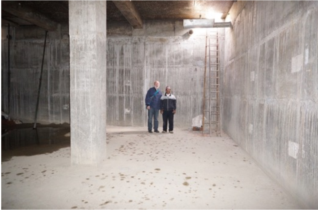
Inside water tank
