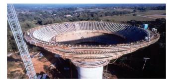
*Fig. 1.4h—Construction of concrete elevated tank (photo courtesy of Crom LLC).*
