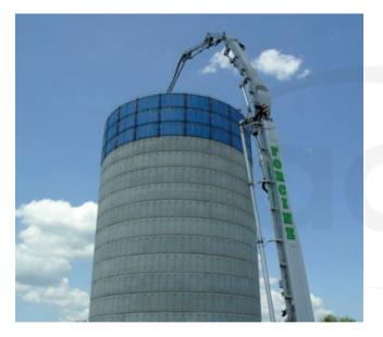
Fig. 1.4g—Construction of composite elevated tank pedestal (photo courtesy of Caldwell Tanks, Inc.).
