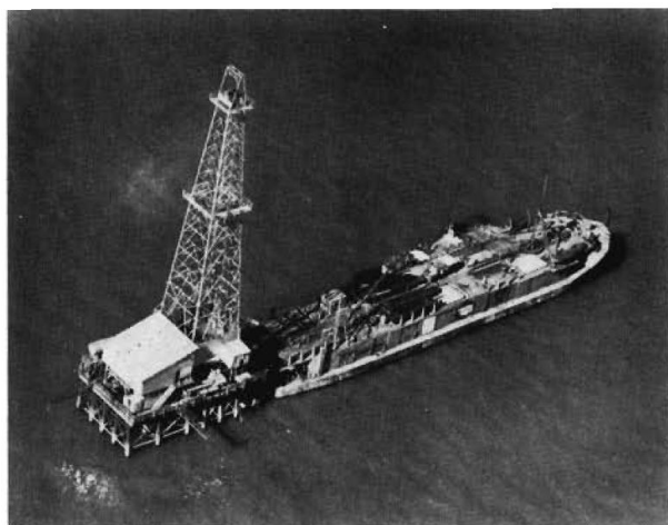
Fig. 1 Small drilling platform with the pioneer floating structure in GoM: an anchored floating tender offshore Louisiana 1) .
