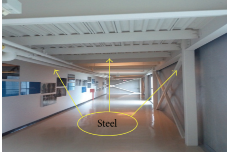
(a) The structure at the CCIT 2nd floor
