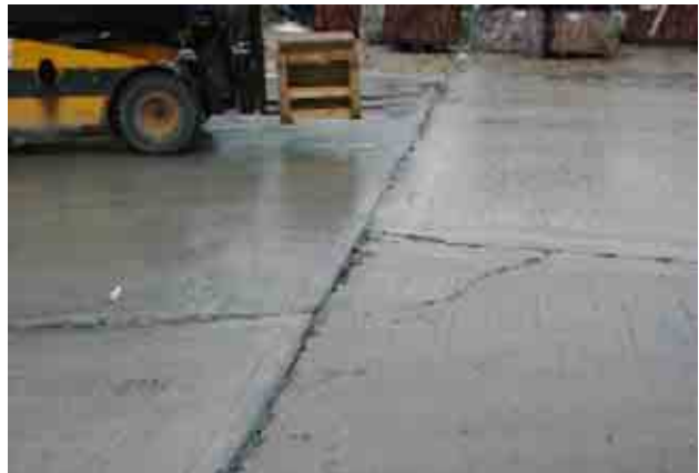
Figure A1.11.2 Operating conditions on Hulland Ward site
