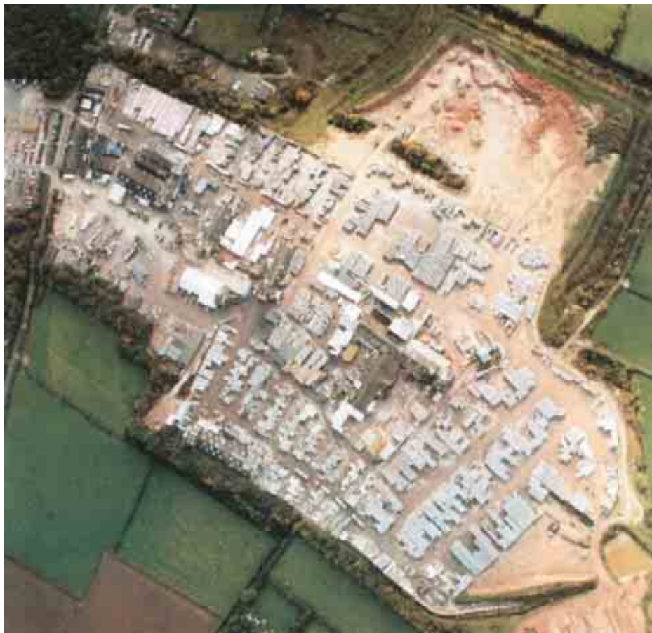
Figure A1.11.1 Aerial view of Hlland Ward site
