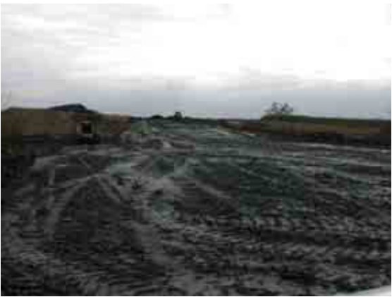
Figure A1.14.1 Site Operation
