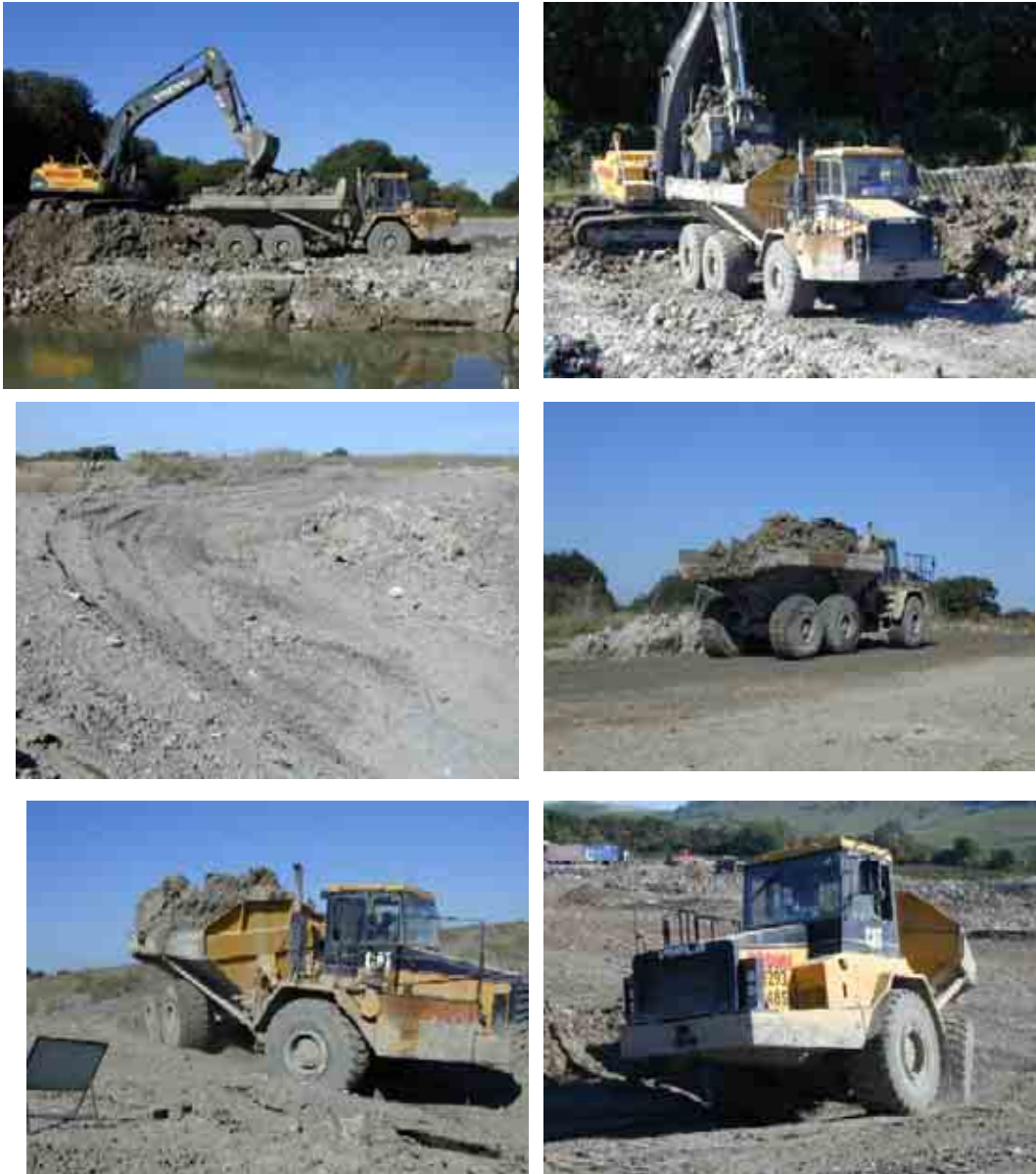
Figure A1.3.1 Caterpillar D250E 25-tonne articulated dump truck at work on-site
