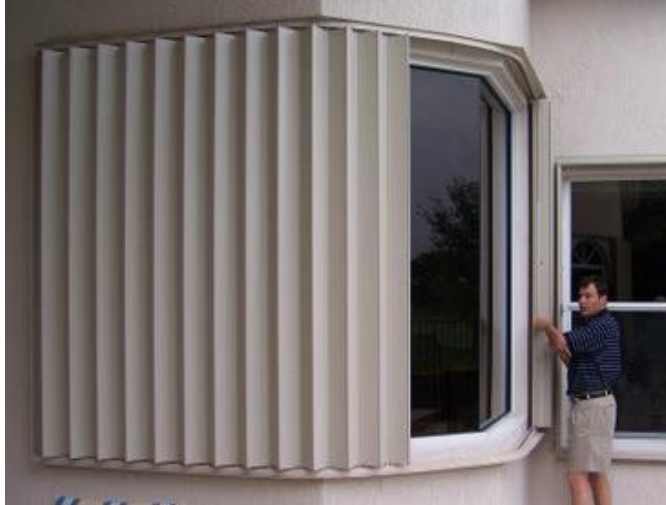
Figure 35: Typical accordion style shutter. Image source: Hurricane Shutters Florida, 2013
