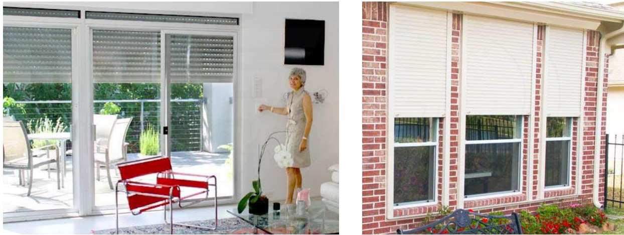
Figure 89: Example of insulated rolling shutter installed on residential building. An interior view is shown on the left, while exterior view is shown on the right. Image source: Rollac, 2013.
