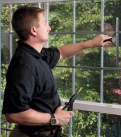
Figure 121: Low-E film on interior glazing. Image Source: Vista Window Film, 2013
