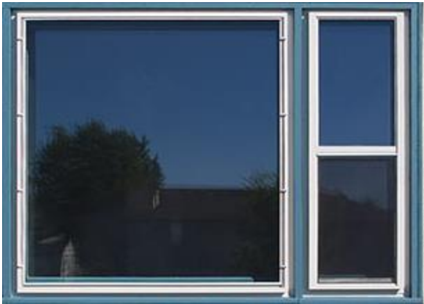
Figure 78: Storm window installed on existing window jamb. Image source: Larson, 2013.
