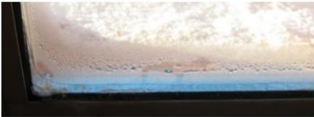
Figure 42: Condensation can easily form on the surface of windows using highly insulative shutter systems. Image source: Craven and Graber-Slaght, 2011.
