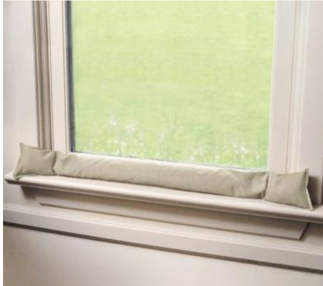
Figure 124: Draft Snake on window sill. Image Source: This Old House, 2013.
