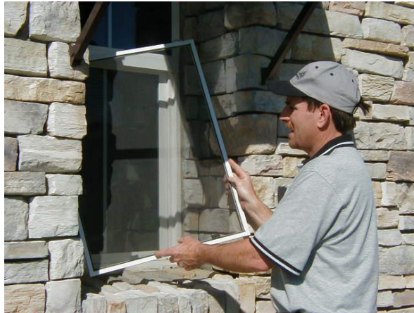
Figure 110: Insect screens, with their fine mesh, provide shading on the window. Image Source: Screen Mobile, 2013
