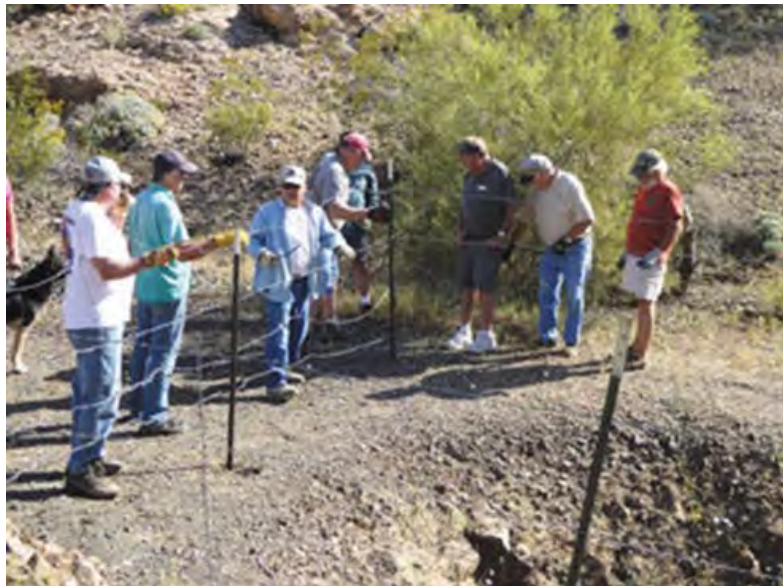
Darryld Kautzmann & crew fencing off another dangerous mine shaft
