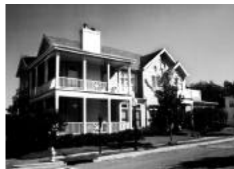
Porches and balconies at Harbortown in Memphis, Tennessee
