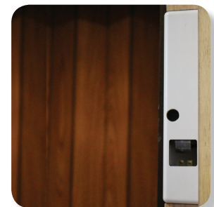
Electro-Mechanical Interlock (EMDL)
