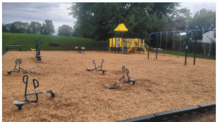
Playground renovation was completed at Miller Park this October.
