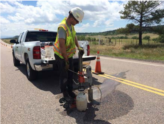
Figure 4. Core sampling
