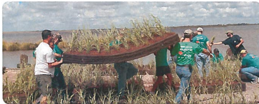
Fig. 8.4 More than 100 Entergy volunteers helped launch floating islands in a demonstration project of a new technology to protect the Gulf Coast south of Houma, La., considered to be ground zero for coastal land loss in America. The floating islands are man-made ecosystems anchored in place in open water that mimic naturally occurring wetlands. They provide nature a starting point to help jump start wetland restoration.
