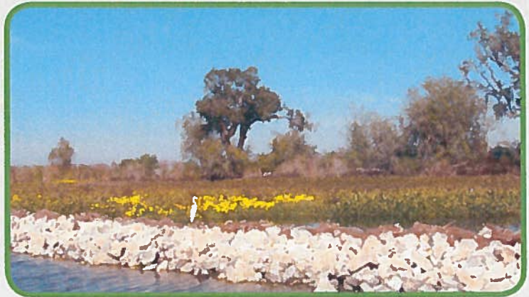
The Bayou Segnette cypress reforestation project in the Barataria Preserve included construction of protective rock jetties to reduce erosion.
