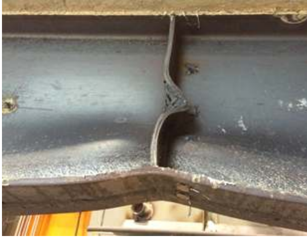
(a) Local buckling of web
