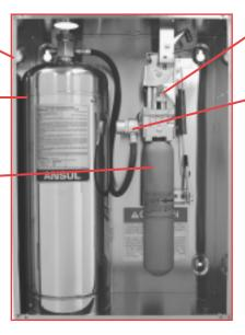
ANSUL AUTOMAN Release... Visible cocked/fired indicator... provides positive actuation of system... needs no periodic adjustment.
