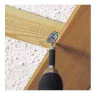
Step 3 Install planks with appropriate clips
