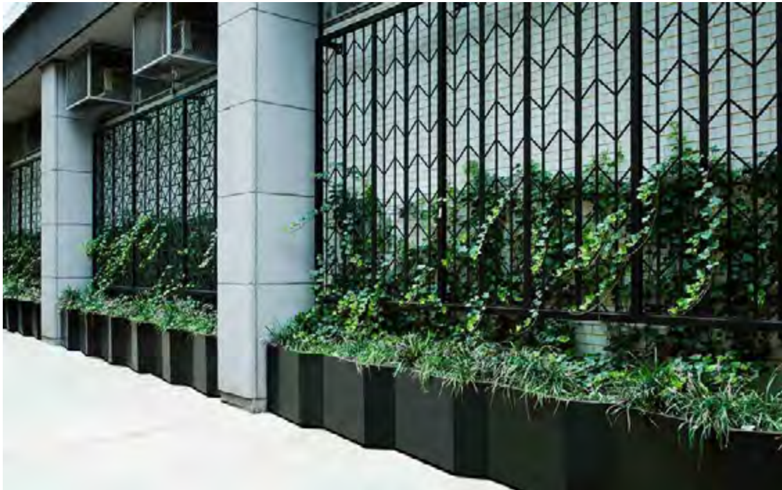
Screen and planters along the back side of the store both conceal mechanical elements and add visual interest to the long bare wall.
