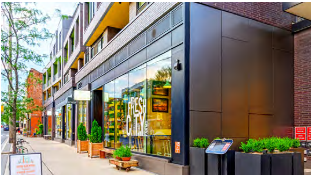
Venting and other base building services integrated into the base building frame around the façade.
