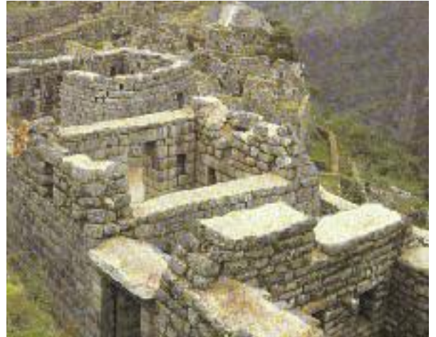
Mortarless construction has been used for centuries.
