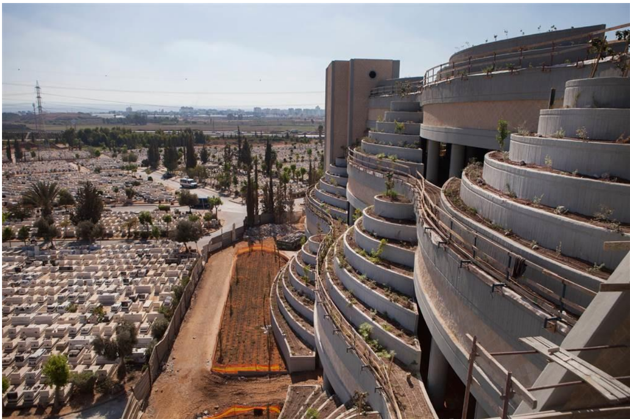
Figure 4–10: The nearly completed vertical cemetery looms over its predecessor Source: (Balilty, 2014)
