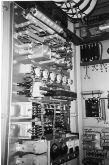
Figure 9: Underexcited Reactive Ampere Limit panel
