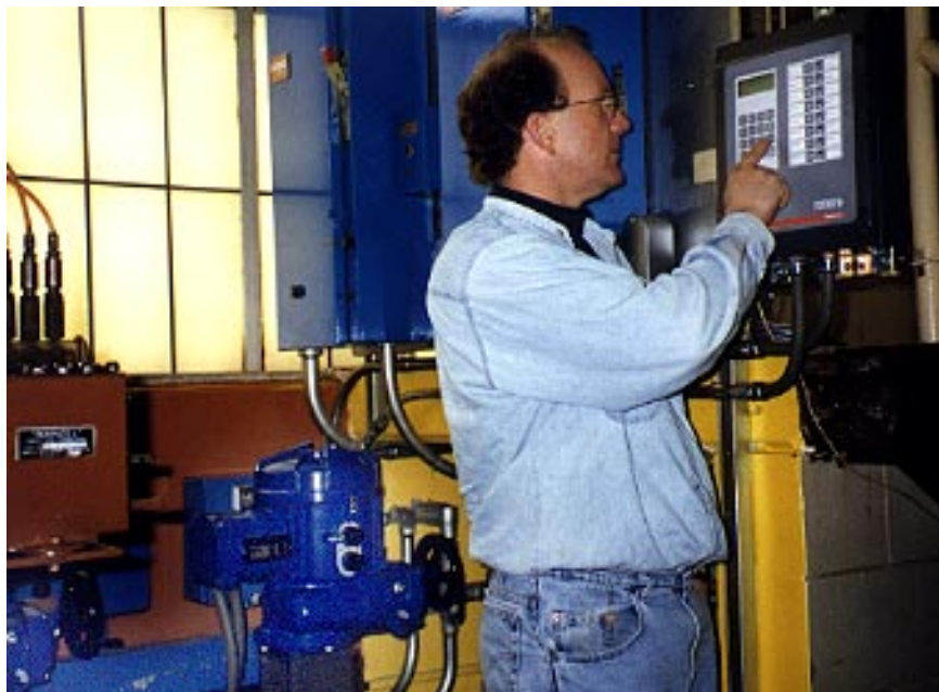
The Pakscan IIS two-wire communication system offers a cost-effective way for water and wastewater treatment plants to obtain the benefits of valve automation. An AQ actuator is pictured in the background, and a programmable Pakscan IIS master station is at top right.
