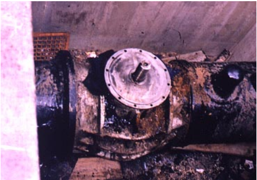
Pictured above is a valve topworks flange and stem onto which an adaptor and actuator will be mounted for a successful retrofit.
