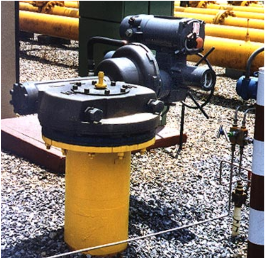
The photograph above shows an example of an A Range actuator plus quarter-turn gearbox.
