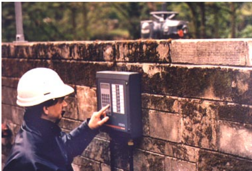
The Pakscan IIS master station is water-tight and can be located indoors or outdoors.
