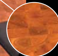
For the Rothwell Recital Hall flooring, designers chose mesquite wood for its beauty and unique end grain cut as well as its enduring quality in combating wear and tear.
