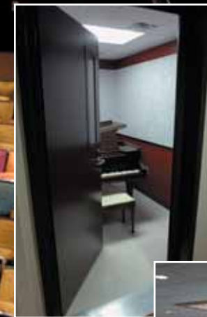
Normal walls are 4 3/4 inches thick. Most walls in the building are now 15 inches thick, with layers of gypsum board, sound insulation and air space. The majority of doors used in the building are high-tech, specialized doors for soundproofing.
