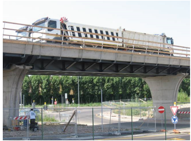
FIGURE 12: Testing of a bridge.
