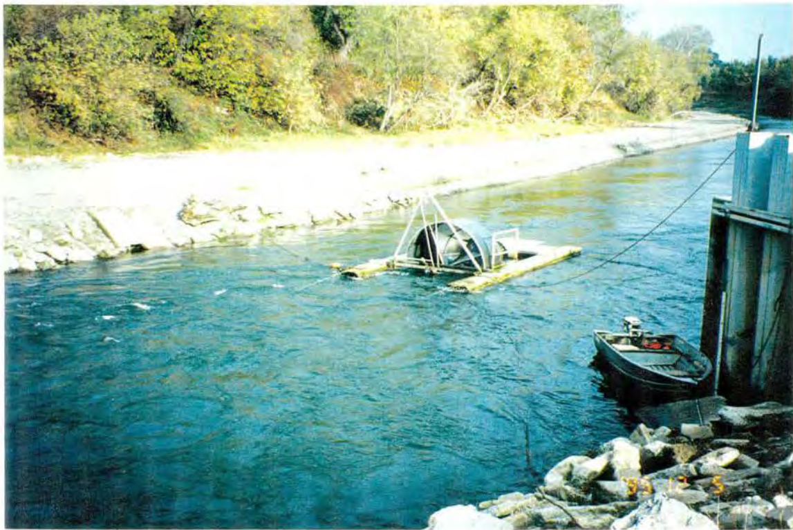
Photograph 12. - Glenn Colusa pumping plant bypass flow (note fish trap).
