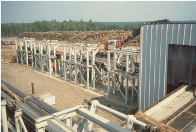
Figure 20—After it leaves the bucking station, pulpwood is routed by chain conveyor to the satellite chipmill (left). Cross-tie logs and sawlogs are transported to the grading station by transverse chain (building on right). Logs are then sorted by product into four sorts where a hydraulic loader bunches logs for transport for loading or temporary storage. Photo taken from the operator's station.
